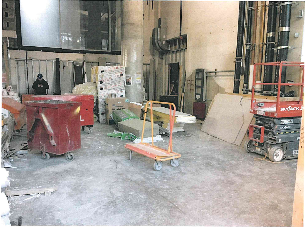
First floor lobby, east
