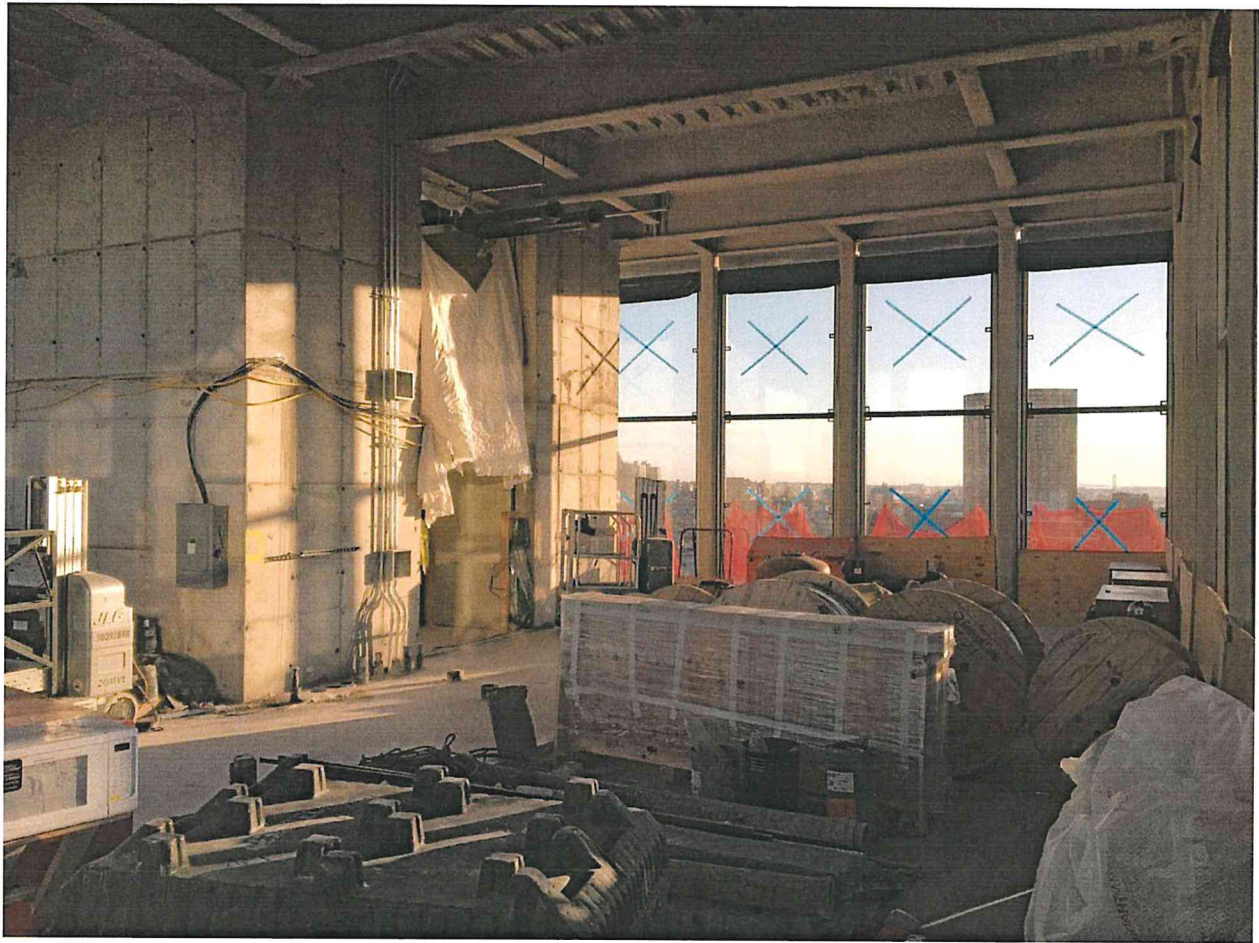
cloudM interior, south
