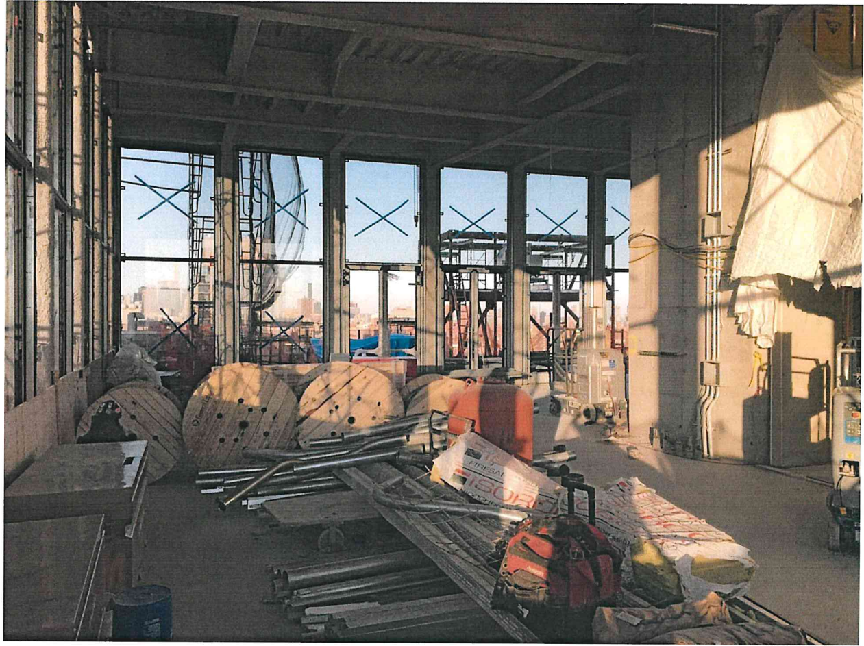
cloudM interior, north
