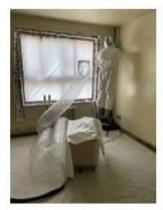
Abatement worker applying peel-away. Mechanical ventilation system in use. (Building 2 – 210K W 153<sup>rd</sup> St,
