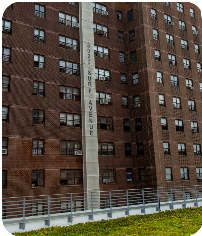
Natural gas conduits, different design solutions: Blue conduit enclosures in Ocean Bay Bayside (bottom left), Exposed conduits in Gowanus (top left), Brick color enclosure in Smith houses (top right), Contemporary enclosure and reuse of existing conduit in Coney Island Houses (bottom right)
