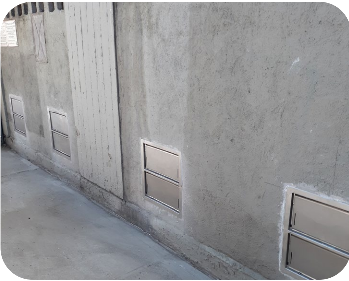
Two Bridges: wet floodproofing vents seen from the outside of the building
