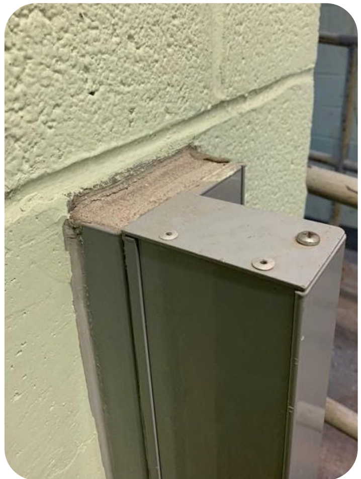
Two Bridges: in order to protect a fire pump room, a deployable flood barrier is installed inside the building
