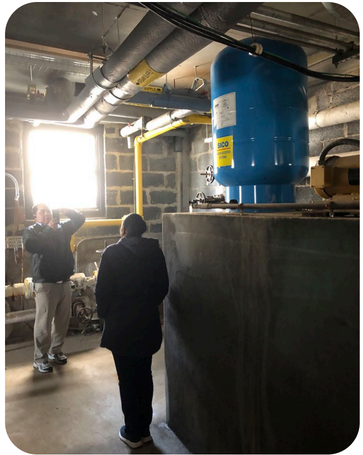
Raised equipment at Ocean Bay Oceanside
