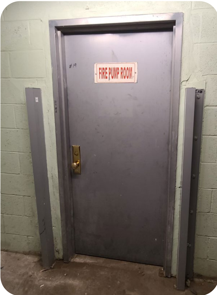
Two Bridges: in order to protect a fire pump room, a deployable flood barrier is installed inside the building
