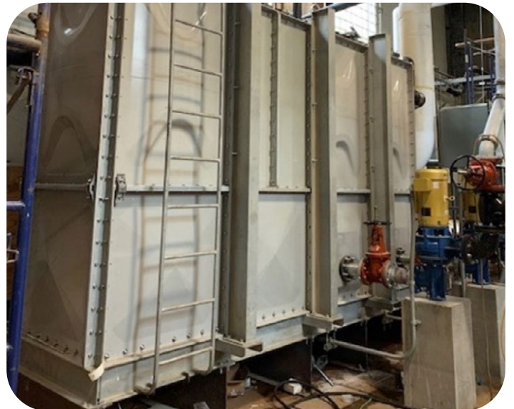
Coney Island Houses: reinforced wall (left) and sum pumps (right) in the basement that need to be protected from flooding.
