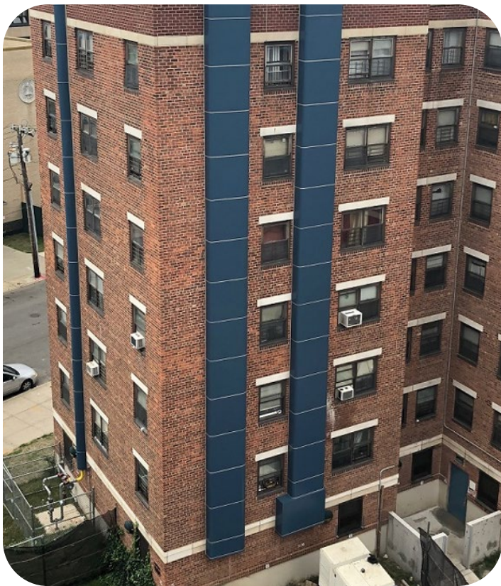
Natural gas conduits, different design solutions: Blue conduit enclosures in Ocean Bay Bayside (bottom left), Exposed conduits in Gowanus (top left), Brick color enclosure in Smith houses (top right), Contemporary enclosure and reuse of existing conduit in Coney Island Houses (bottom right)
