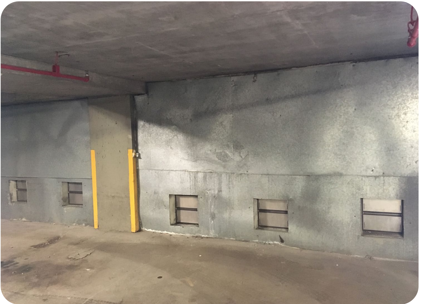
Two Bridges: the parking area has vents in order to wet floodproof
