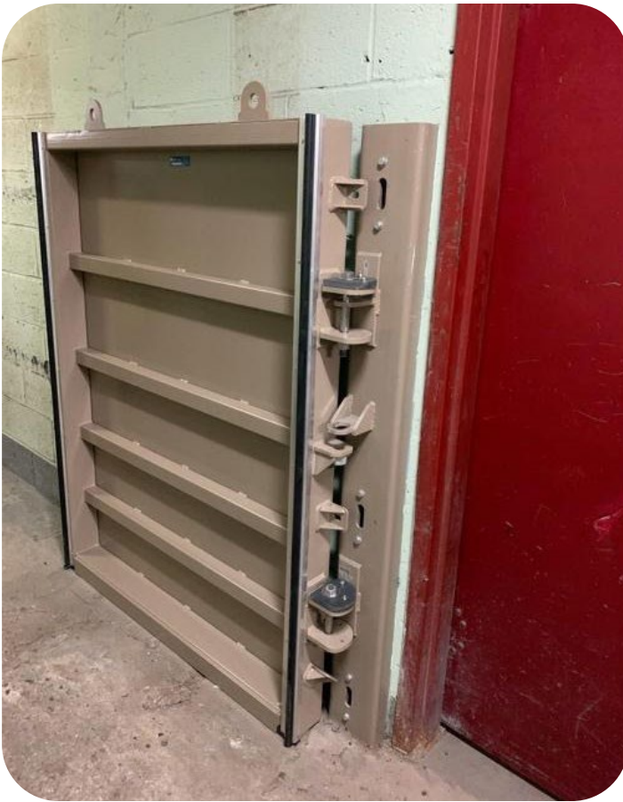
Two Bridges: Flood door in a hallway in the basement to delineate a protected zone
