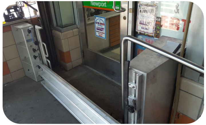
Lower East Side V: Deployable flood panels in front of a store
