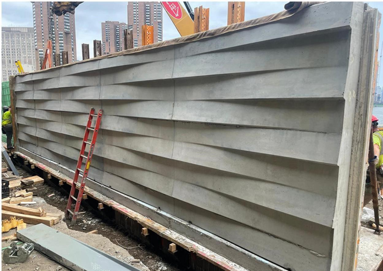
Figure 7: East Side Coastal Resiliency Section of Floodwall Under Construction
