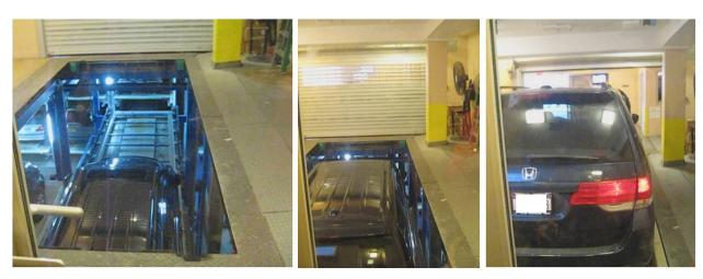
Figure 8 Automated vehicle retrieval in 123 Baxter facility
