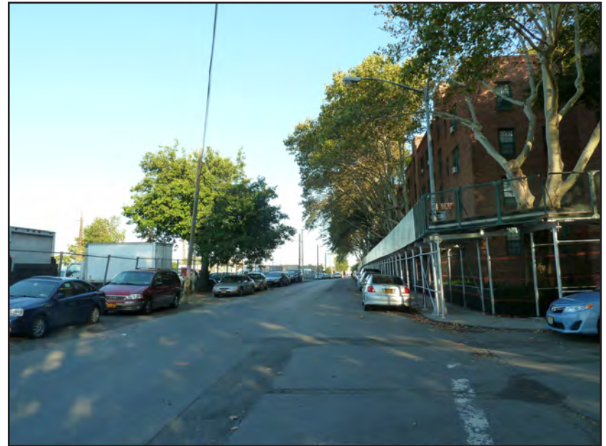
4. View east from northwest corner of 50th Street and Barnett Avenue.
