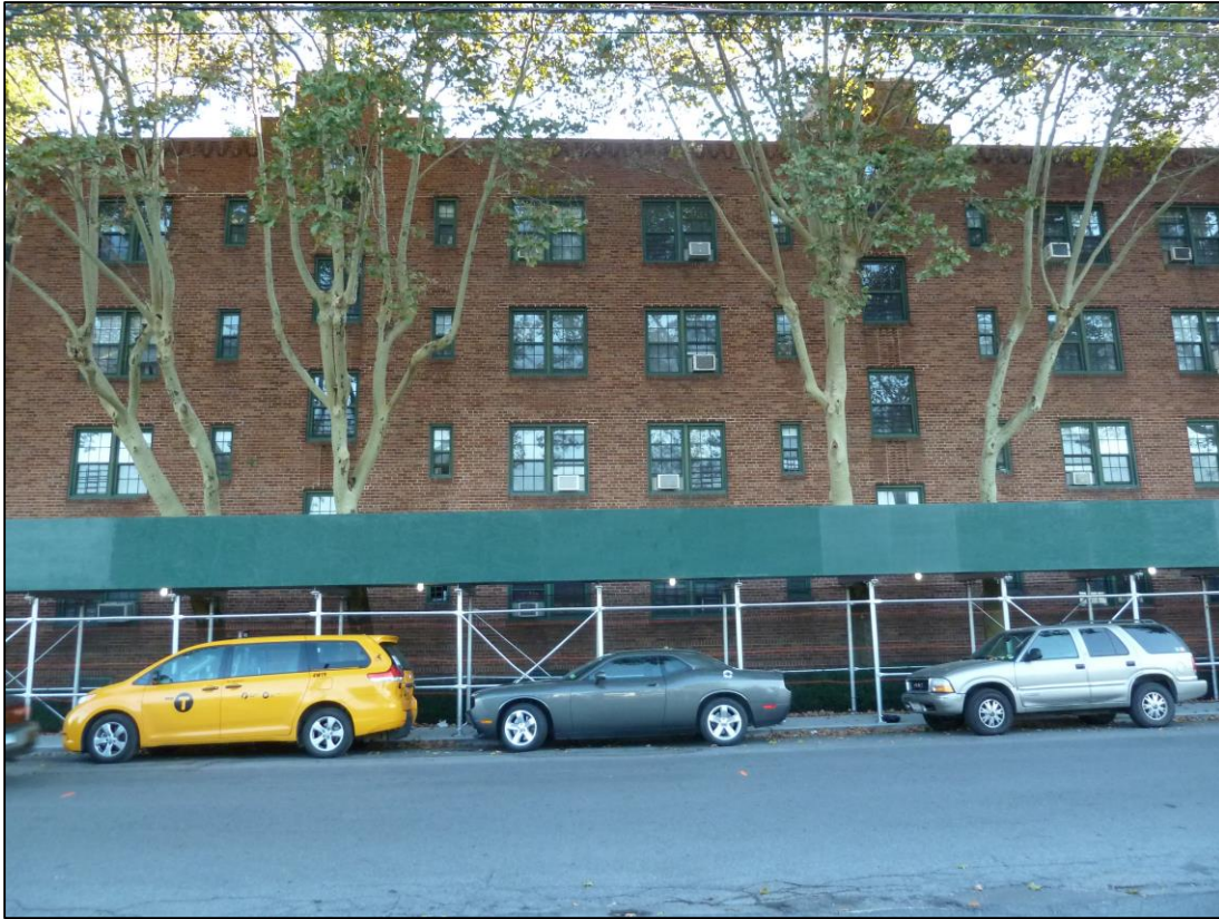
View south of Phipps Garden Apartments II (north façade) from the southern border of the primary study area.
