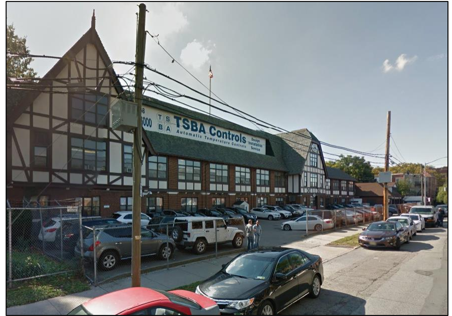
View southwest of mixed-use office/light industrial building at southwest corner of Barnett and Woodside Avenues
