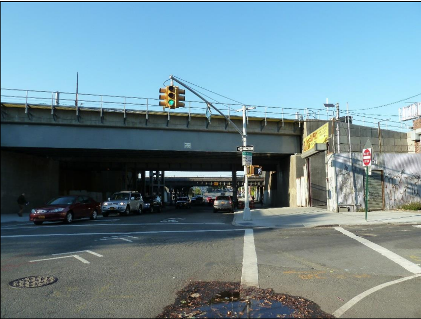
View north from southeast corner of Barnett Avenue & 48 th Street
