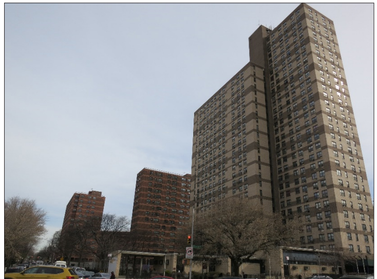
Atlantic Terminal complex, view northeast from Carlton Avenue 12
