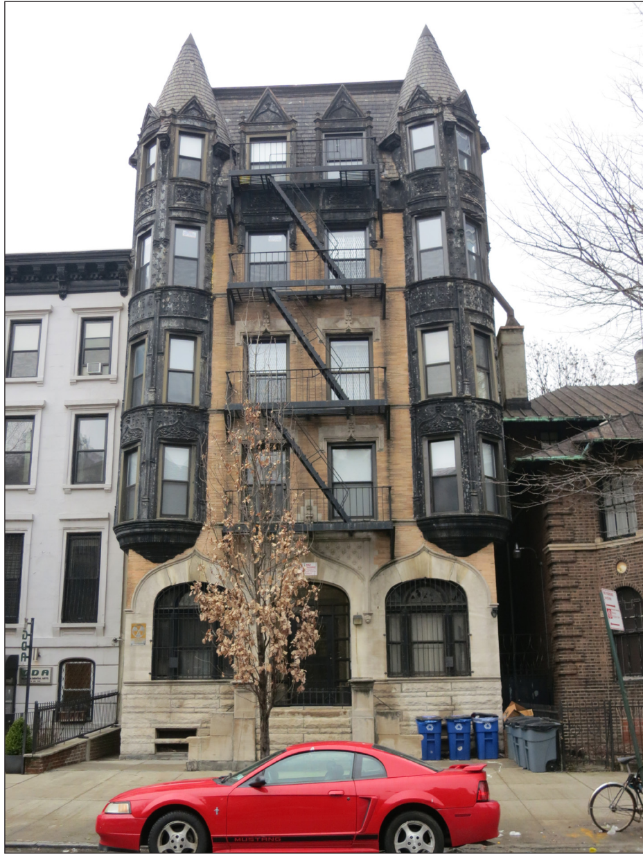
View east of the western (front) façade of the apartment building at 515 Clinton Avenue 7
