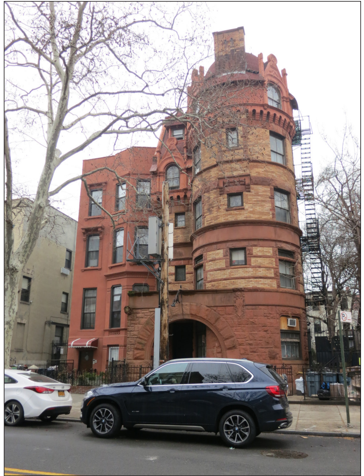
View east of the western (front) façades of 483 Clinton Avenue and 487 Clinton Avenue 8
