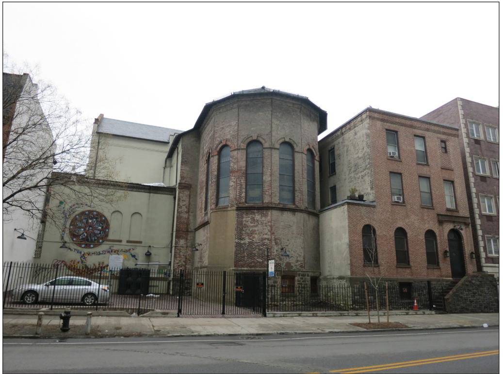
View southeast along Vanderbilt Avenue of the rear façade of the Church of St. Luke and St. Matthew 2
