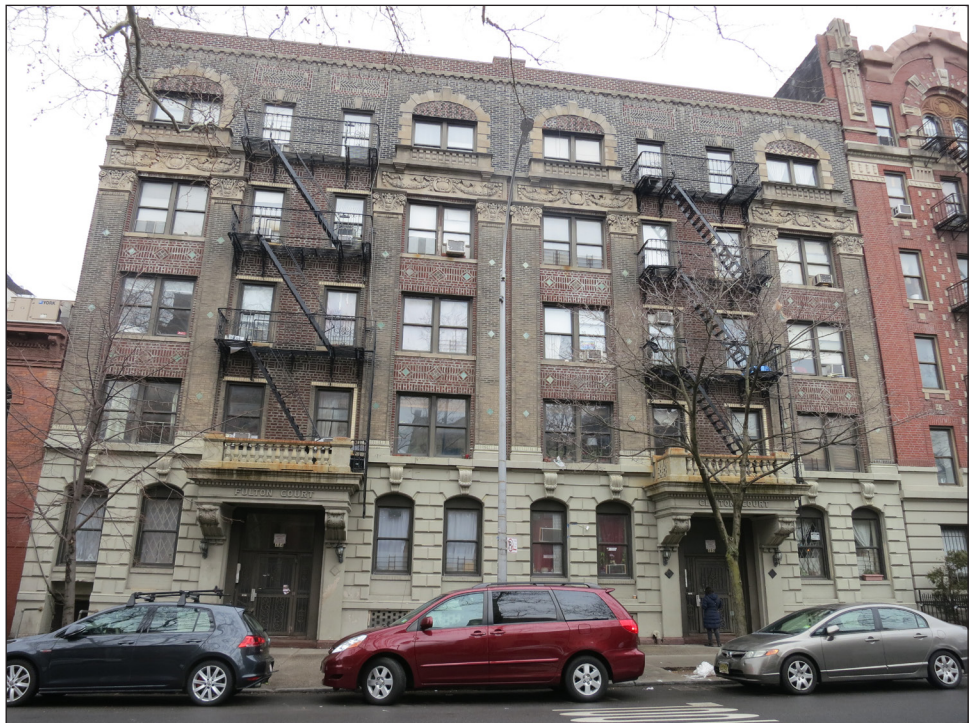
View west of the Fulton Court Apartments (484 Clinton Avenue) and Clinton Court Apartments (480 Clinton Avenue) 9
