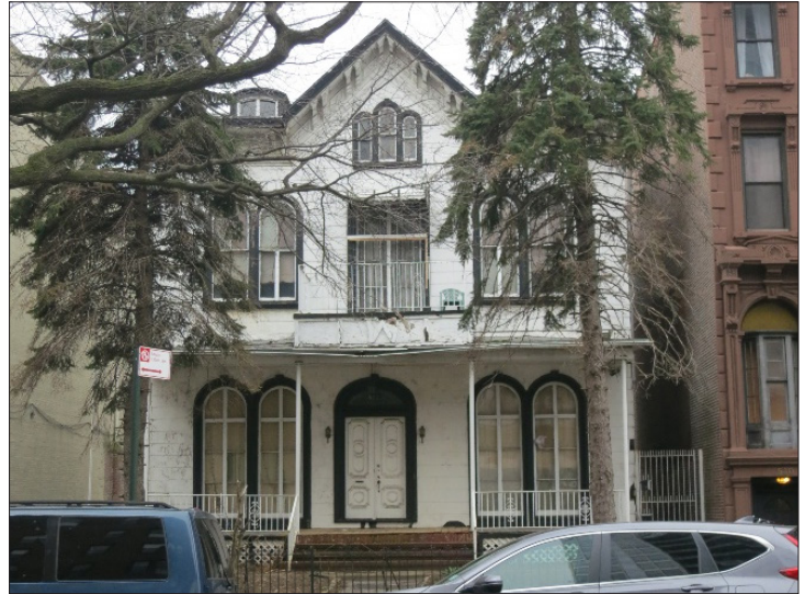
532 Clinton Avenue within rezoning area 7
