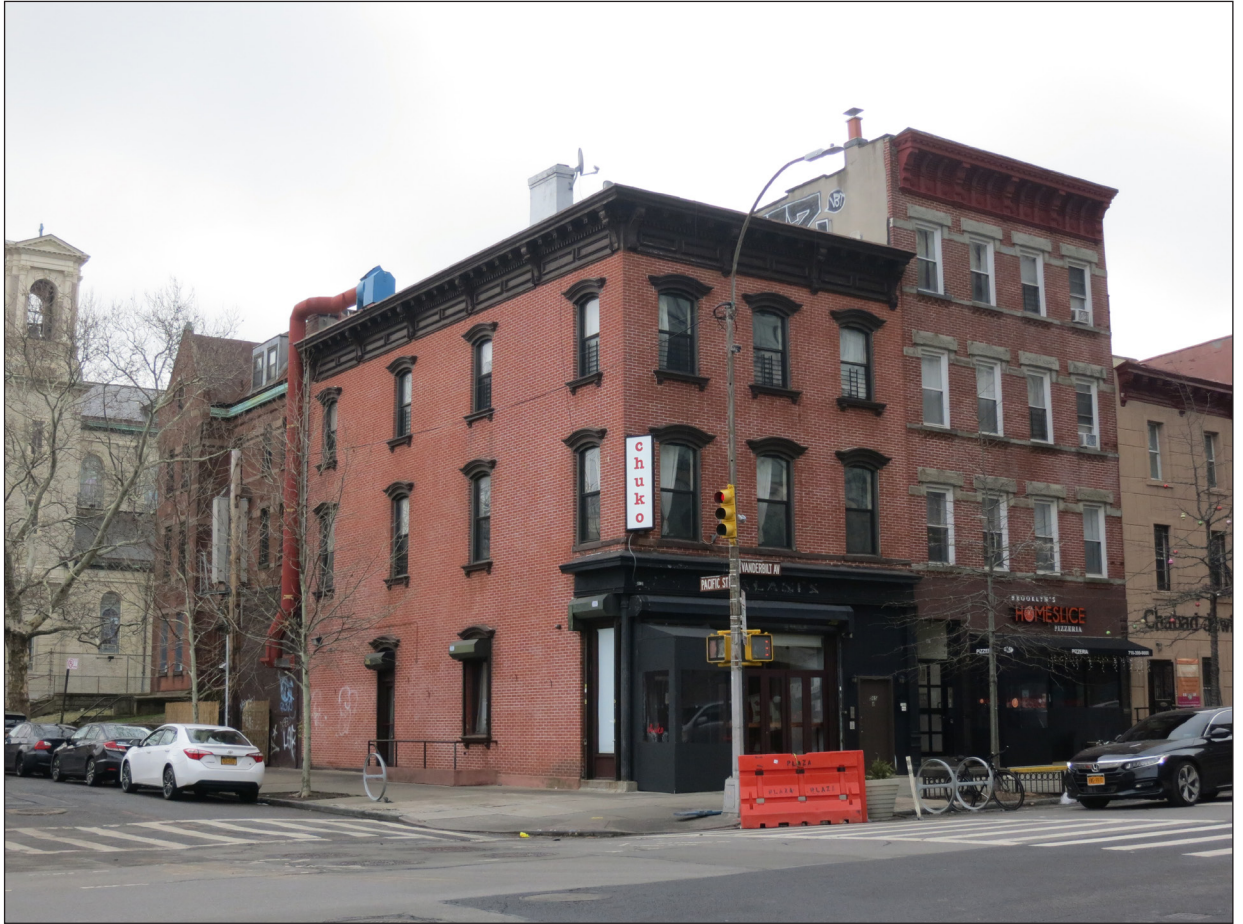
View southeast from the intersection of Pacific Street and Vanderbilt Avenue of the northern end of the Prospect Heights Historic District along Vanderbilt Avenue 10
