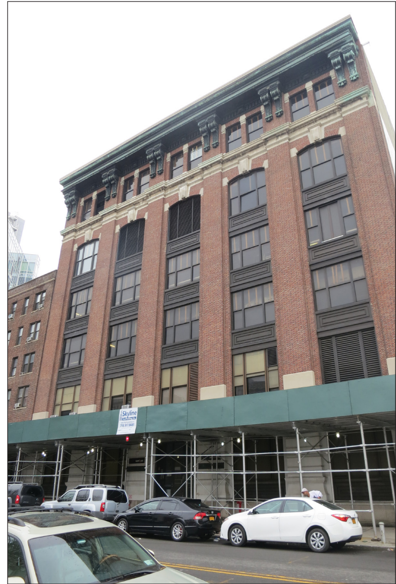
View northeast of the western (front) façade of the old telephone building at 547 Clinton Avenue (S/NR-eligible) 6
