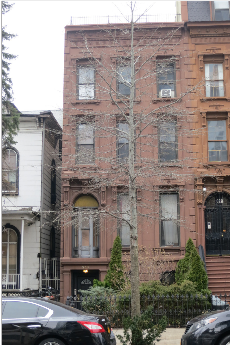
View west of the eastern (front) façade of 530 Clinton Avenue 5
