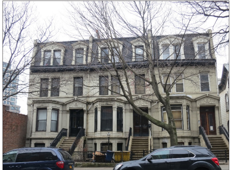
536-540 Clinton Avenue within rezoning area 8
