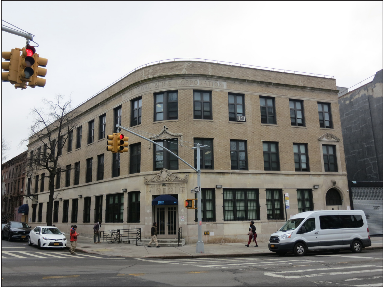
View northeast of 937 Fulton Street from the intersection of Fulton Street and Waverly Avenue 15
