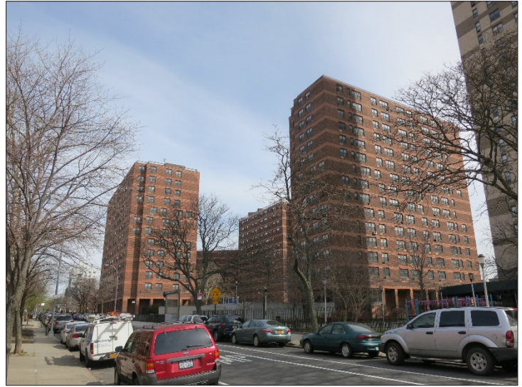
Atlantic Terminal II complex, 13 view northeast from Carlton Avenue
