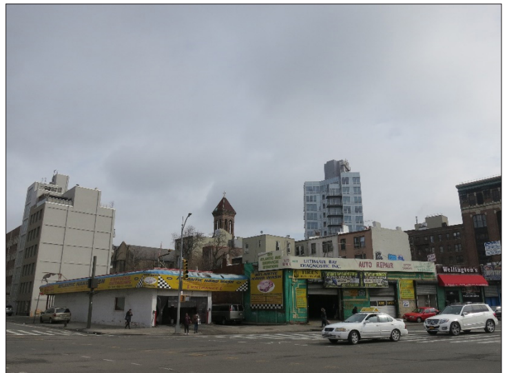
Development site, view northeast from Atlantic Avenue 3
