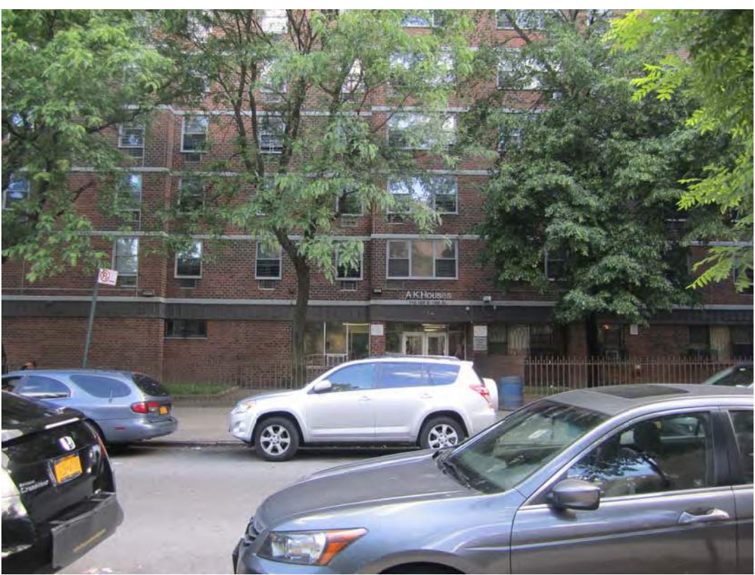
② VIEW LOOKING SOUTH FROM E 128 ST
