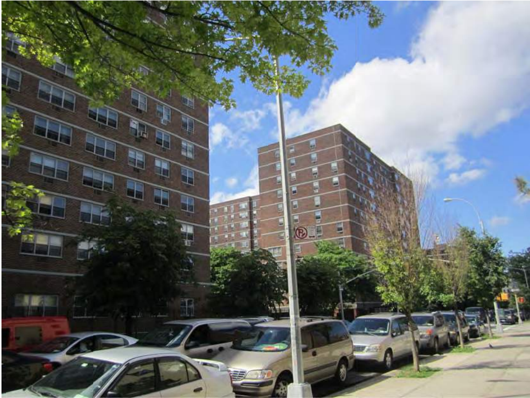
③ VIEW LOOKING NORTHEAST FROM LEXINGTON AVE
