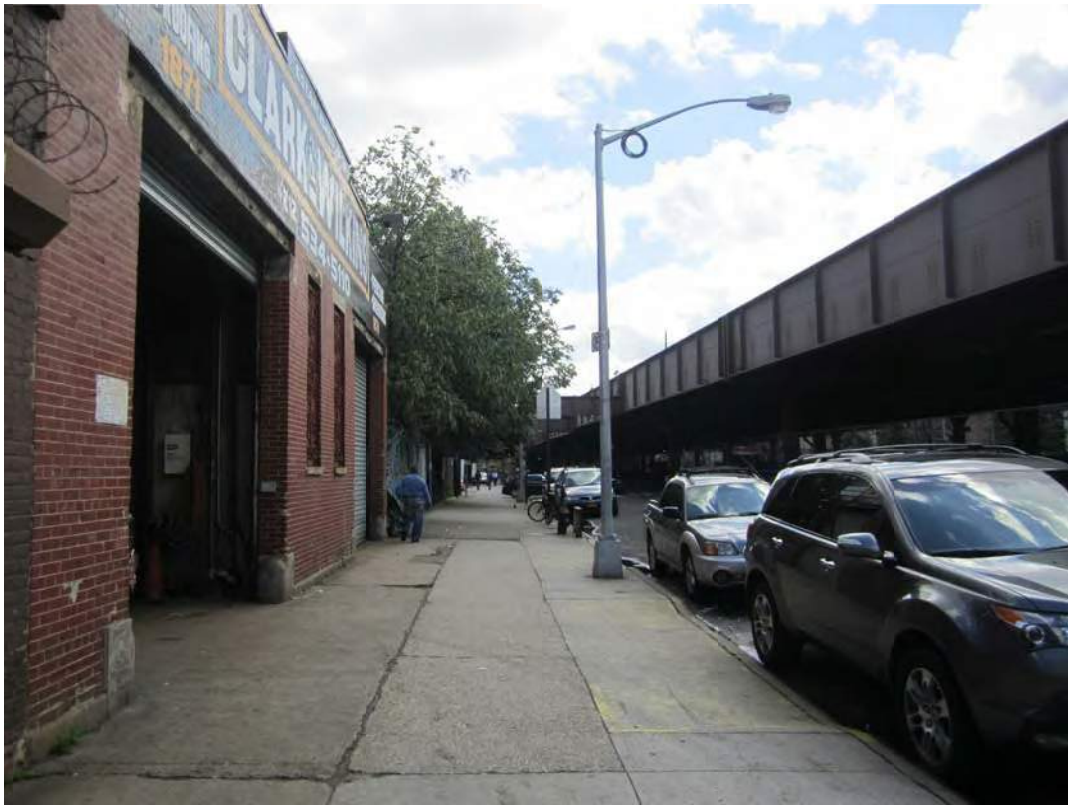
② VIEW LOOKING SOUTH FROM PARK AVE
