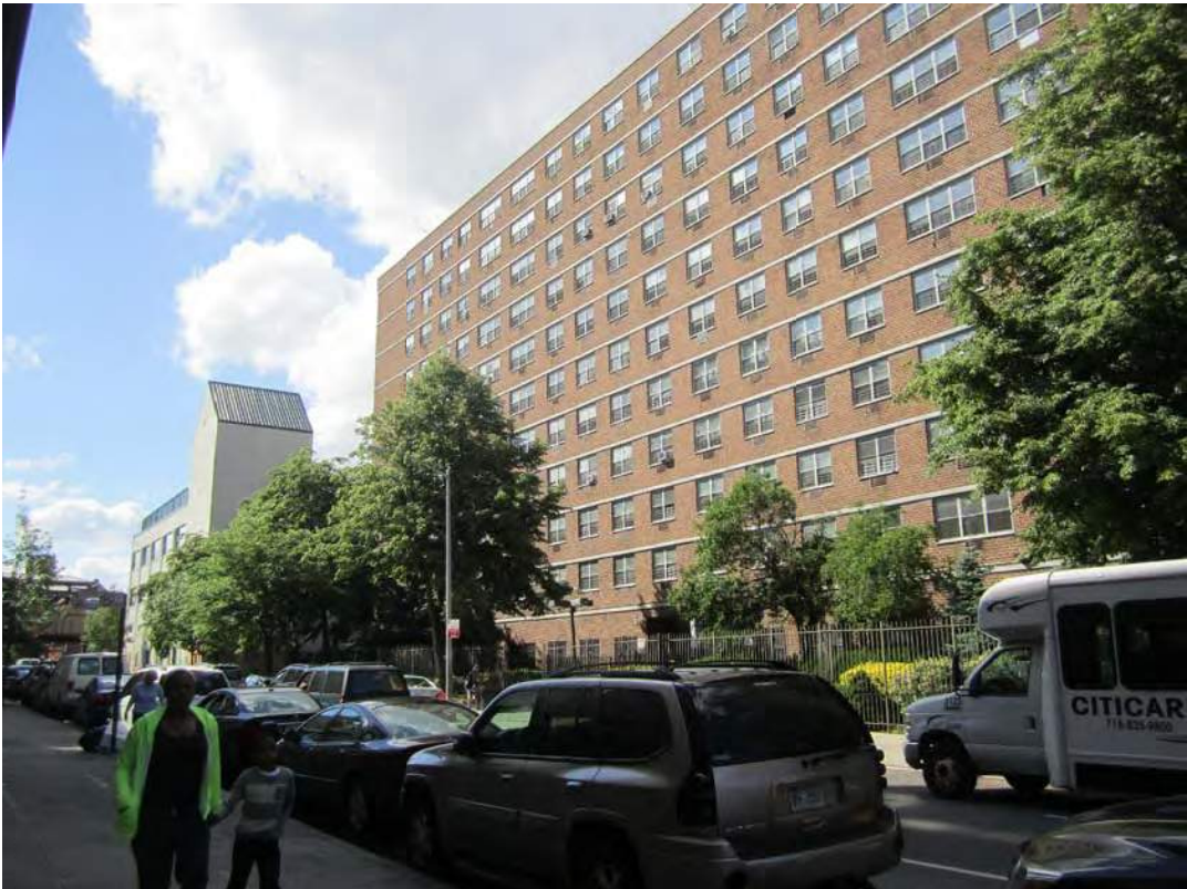
④ VIEW LOOKING WEST FROM E 126 ST AND LEXINGTON AVE
