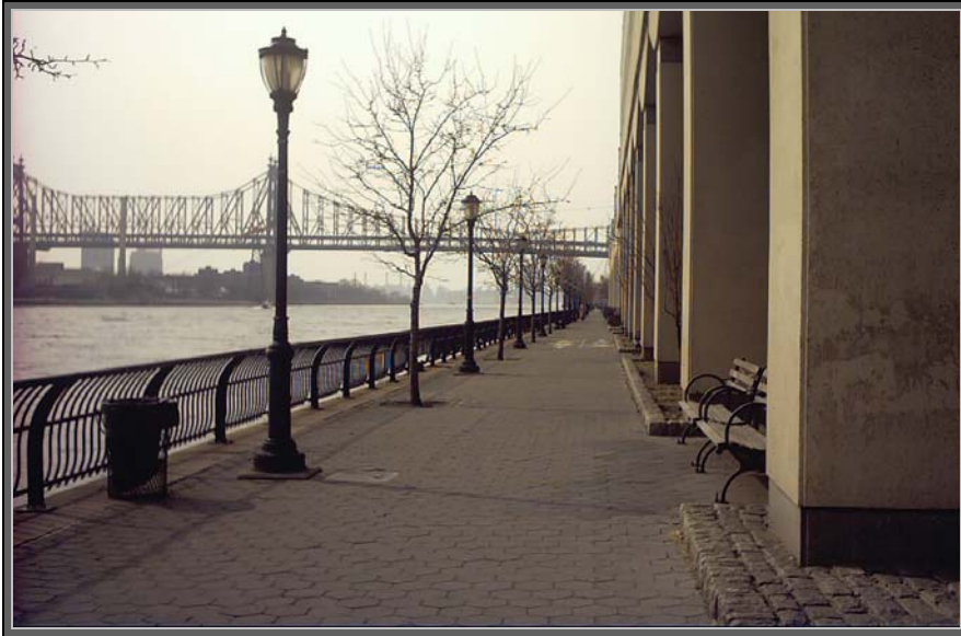
5. View looking south along the esplanade showing footing columns for the East Wing.
