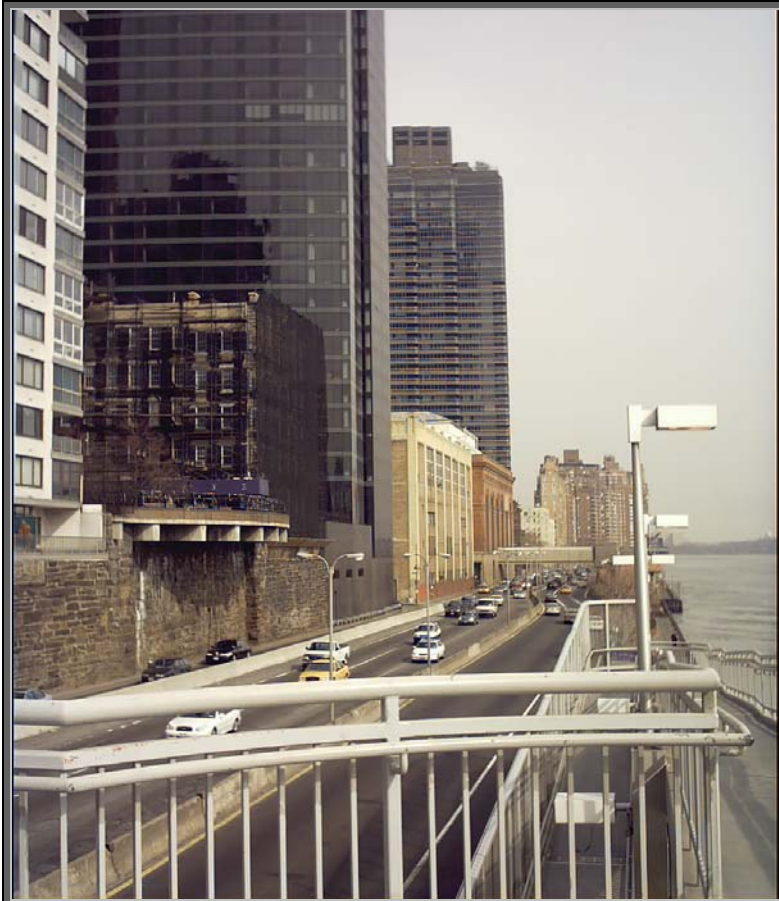
6. View looking north along the FDR Drive from the public pedestrian bridge.
