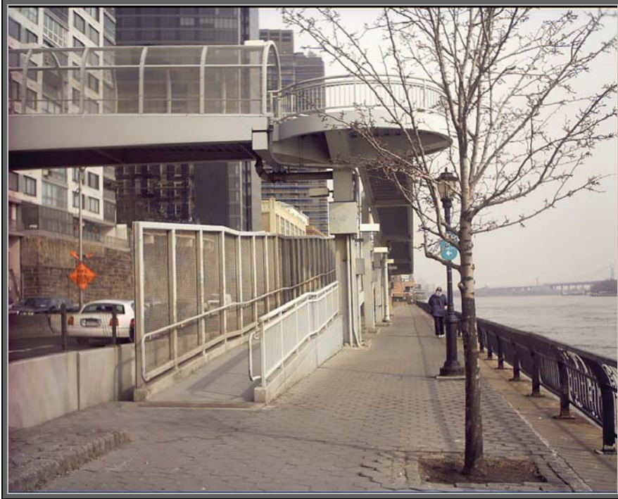
1. View looking north along the esplanade.
