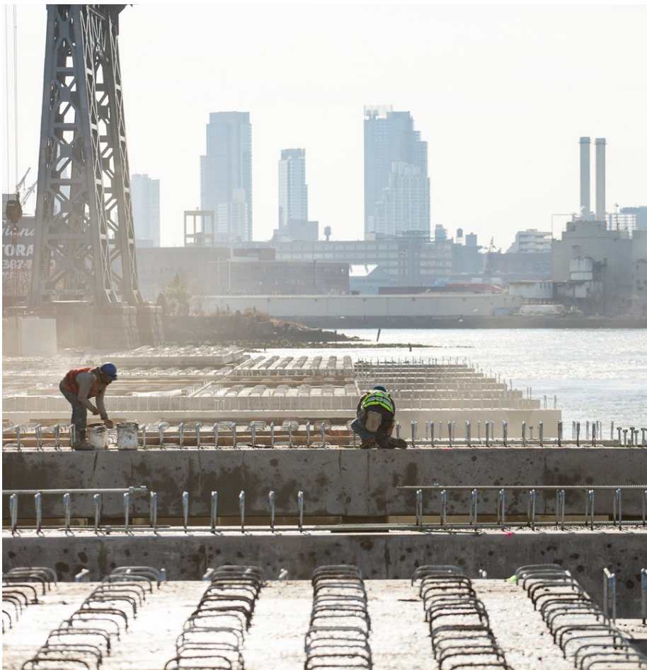
Constructing Domino Park, Brooklyn.
