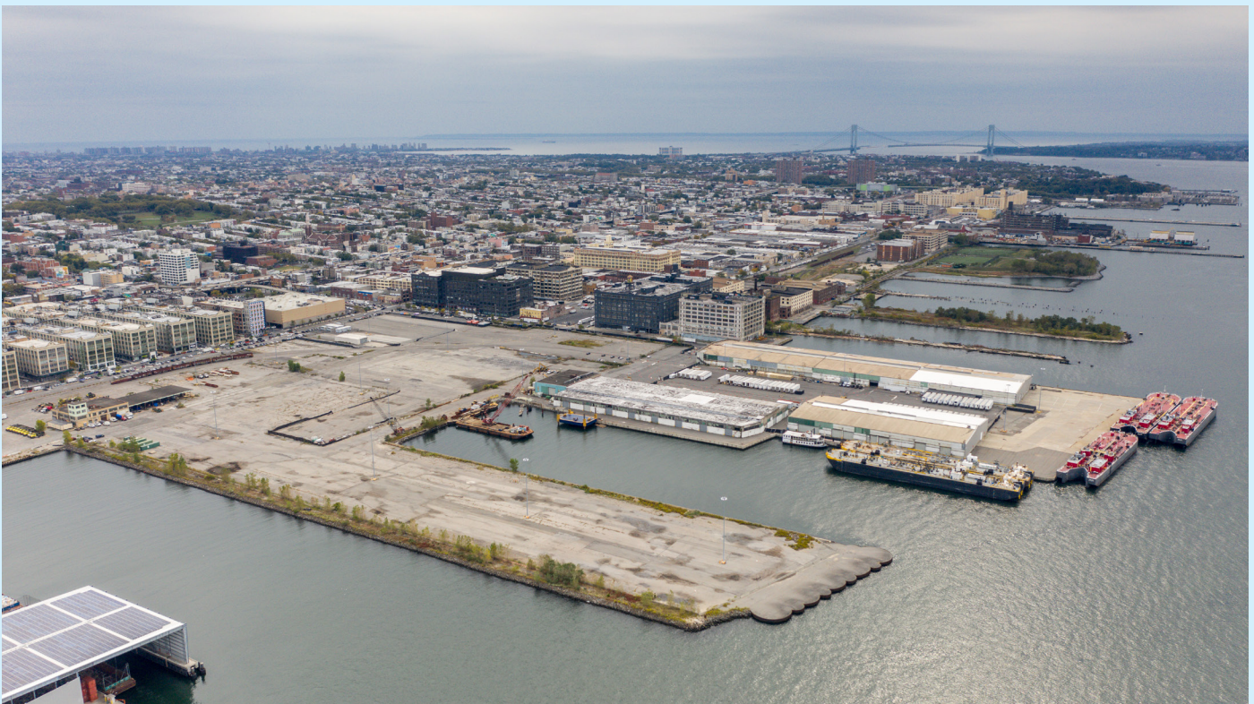
South Brooklyn Marine Terminal. Credit: Sustainable South Brooklyn Marine Terminal
