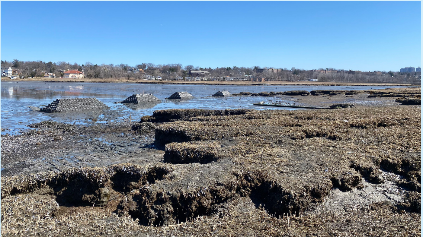
Above: Alley Creek living shoreline installation, Queens.
