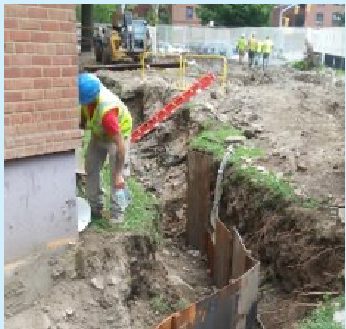
Passive impermeable barriers below grade stop water infiltration and protect building foundations. This photo shows flexible liners being installed below grade at Wald Houses in Manhattan. Credit: NYCHA
