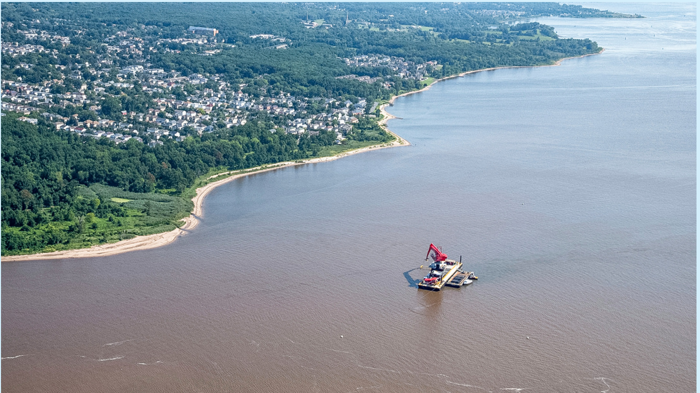
Above: Living breakwaters construction, Staten Island.
