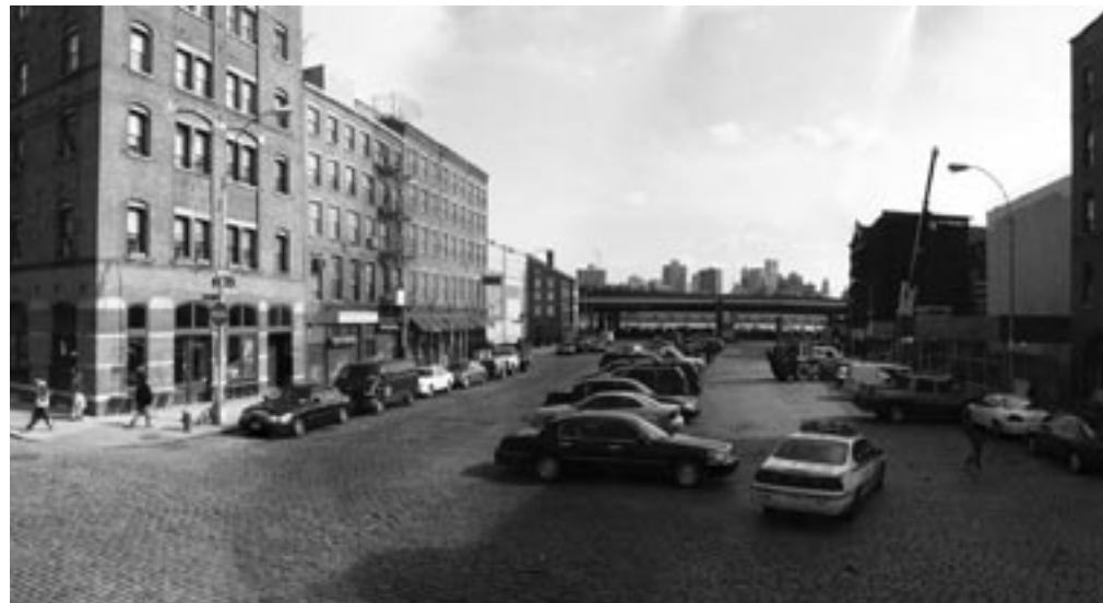
PECK SLIP - EXISTING CONDITION
