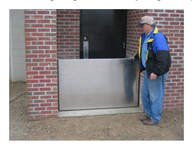
**Deployable floodgate** (currently allowed only at doors and operable windows)
