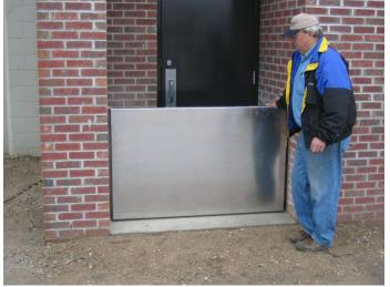
Deployable floodgate (currently allowed only at doors and operable windows)
