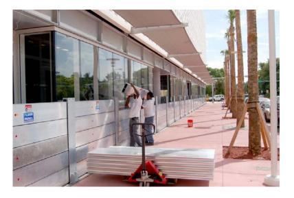
**Deployable floodgate**(allowed at perimeter only for pre-FIRM buildings)
