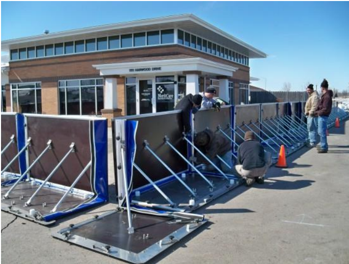
Non-NFIP compliant (e.g. “Aquafence”; allowed for Pre-FIRM buildings)
