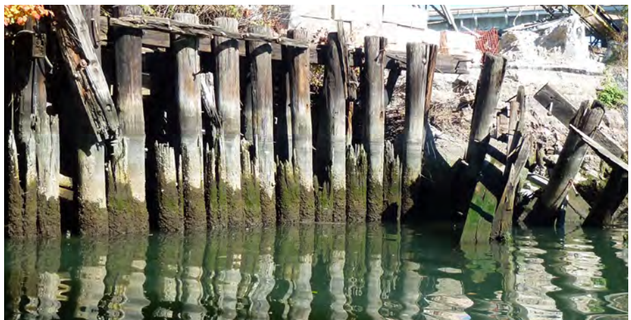
Deteriorating bulkheads
