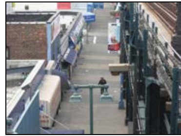
River Avenue, pictured south of 161st Street, is dominated by single-story baseball-oriented uses that remain shuttered on non-game days; the area is currently zoned C8-3.
