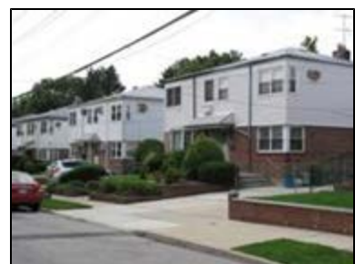
Semi-attached building on 212th Street in a proposed R3-1 district
