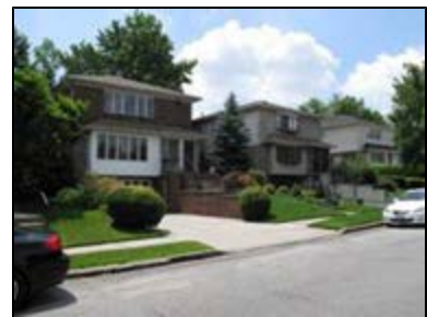
Two family detached homes on 57th Road in a proposed R3X district
