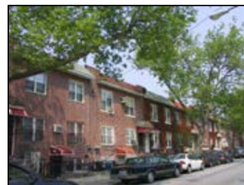
West 7th Street between Avenue S and T - Attached housing in the proposed R5B
