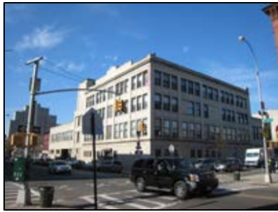
Office Building at 3rd Avenue and Dean Street, Existing R6, Proposed R7A/C2-4
