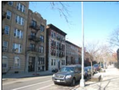
Apartment Buildings on Dean Street, Existing R6, Proposed R6A
