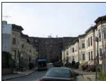
Existing R5: East 8th Street looking towards East 8th Street
