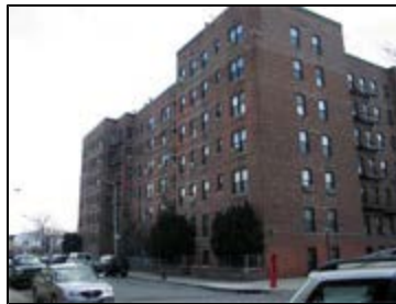
Existing R6: East 8th Street at Kermit Place looking south
