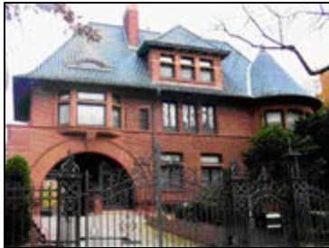
Catholic Bishops Residence, Clinton Avenue
