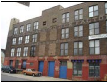
Commercial loft space on Union Street at Nevins Street
