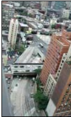
Lincoln tunnel cuts at 9th Ave. and 35th St.
