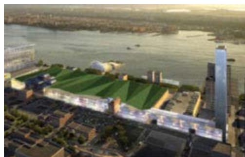
View of Convention Center Expansion, HOK/Kohn Pederson Fox
