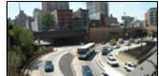
Lincoln tunnel access ramps at 39th Street
