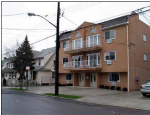
Out-of-context development permitted under existing R5 zoning.
