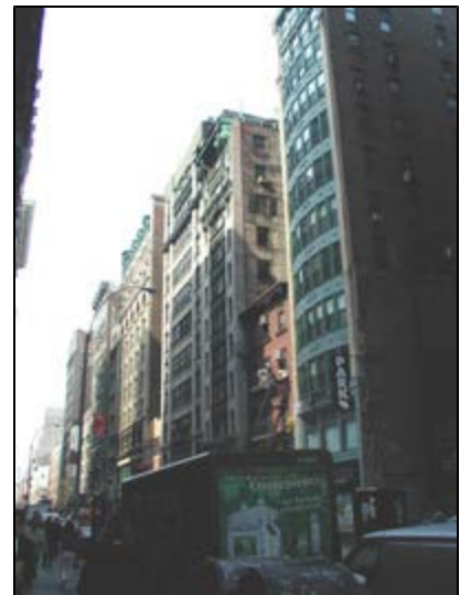
High street wall on north side of 17th Street
