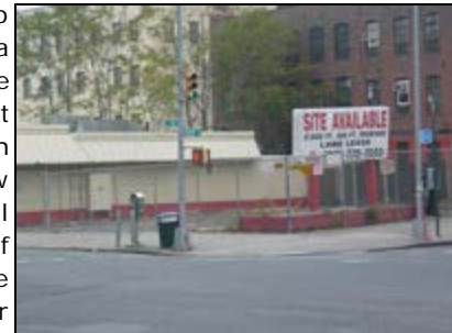
A vacant lot located at 138th Street and Third Avenue in the proposed M1-4/ R7X
