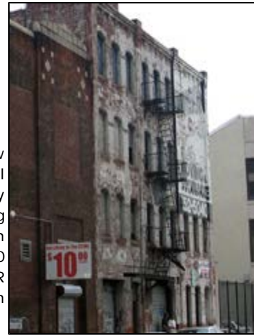
A loft building on Gerard Avenue south of E 144th Street in the proposed M1-4/ R6A
