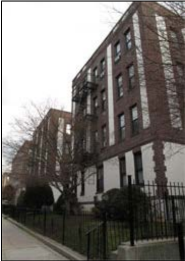
Apartment building at 37th Ave and 168th Street in a proposed R5D district
