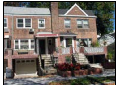
Two-story apartment building on 37th Ave in a proposed R4
