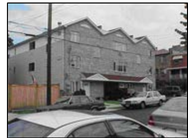
New, out-of-scale construction on Mayflower Avenue in the proposed R5A district
