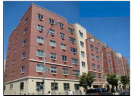
A six-story building along 186th Street in a proposed R6A district.
