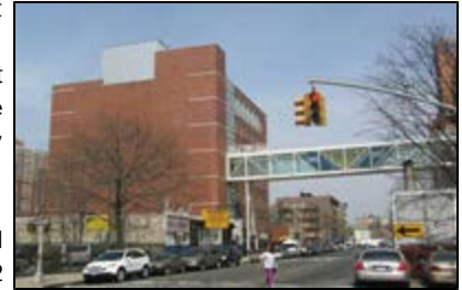
Seven-story St. Barnabas Hospital building along Third Avenue in a proposed C4-4D district.
