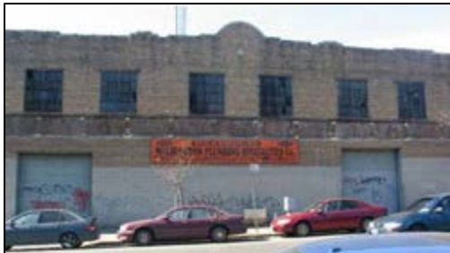
Low scale industrial development, underutilized lots, and parking lots are byproducts of the zoning created for the elevated train along Third Avenue which was removed in 1973.
