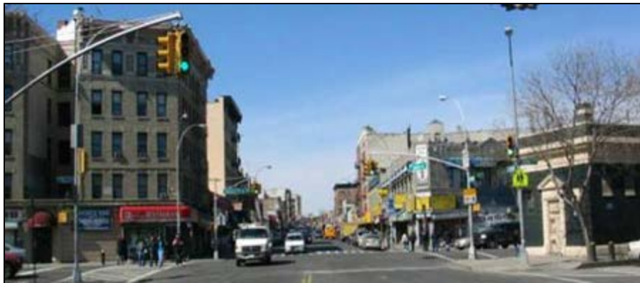
Five-story building on the intersection of Tremont Avenue and Southern Boulevard in a proposed R7X/C1-4 district.
