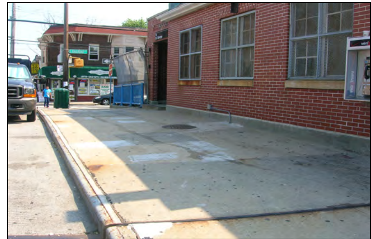
Available space in front of the Grant City rail station to accommodate bicycle parking Grant City rail station
