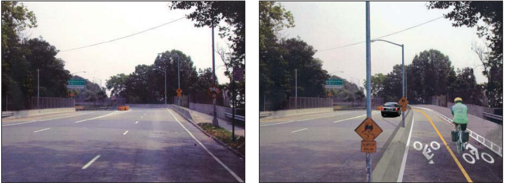
Figure 9: Current conditions and rendering of a reconfigured Highland Boulevard with only one vehicle lane control all traffic, including right turns, at the existing traffic signal [Figure 7]. The crosswalk should be designed for pedestrians and bicyclists and pigmented blue. If necessary, right turns on red could be permitted to enhance traffic movement.
