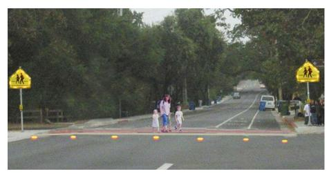
IMAGE 15. Embedded Flashers-The LED flash after the pedestrian enters the crosswalk. Image used with permission from Lightquard Systems, Inc.
