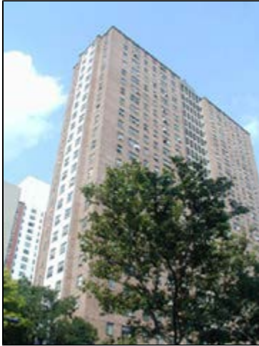
Fulton Houses, West 16th Street between Ninth and Tenth Avenues
