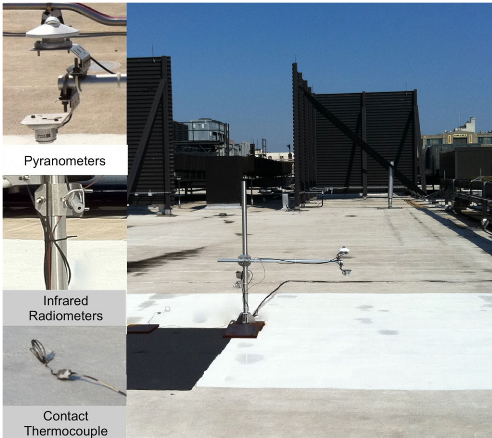
Figure 6.6. Pilot paint program to brighten NYC dark roofs and monitoring sensors. The whitened test surface freshly coated is shown alongside an untreated square of the original asphaltic membrane. The surrounding gray area is the state of the paint two years after an initial coating. (Gaffin et al. , 2012b).
