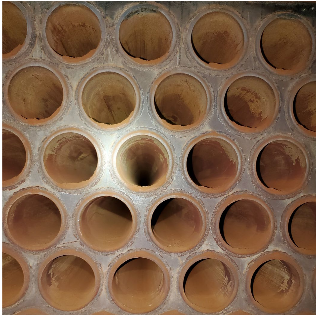
Visual inspection of boiler firetubes
