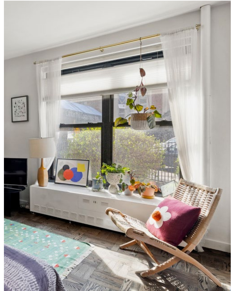
Insulated radiator enclosure
