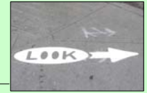
Example: Pavement Marking Warning Message
