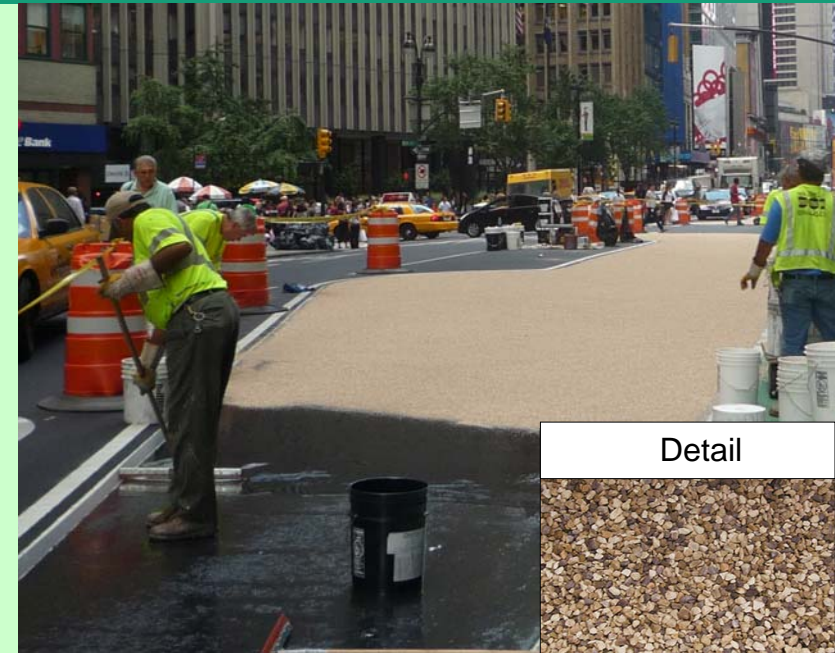
Application of epoxied gravel at pedestrian zone
