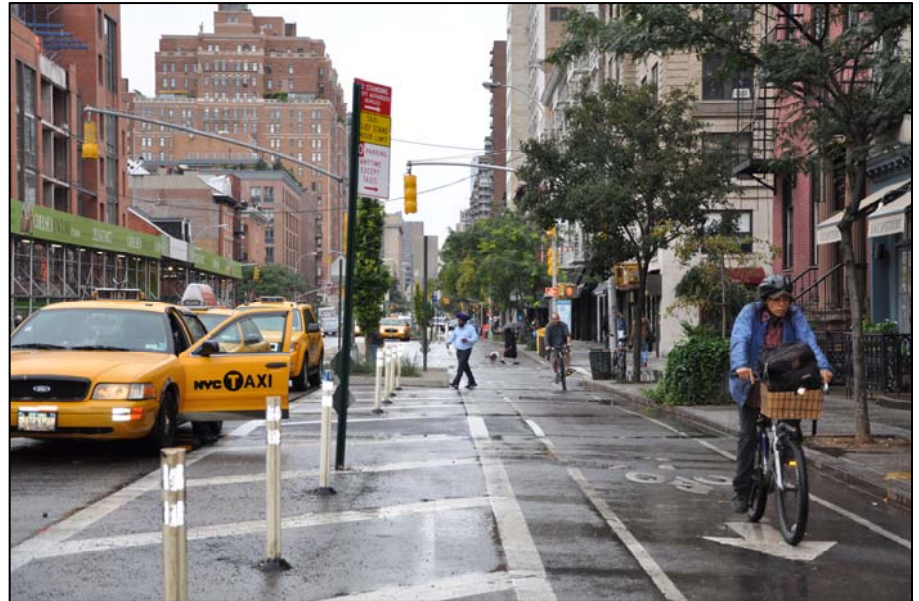
9th Avenue Parking Protected Bike Path
