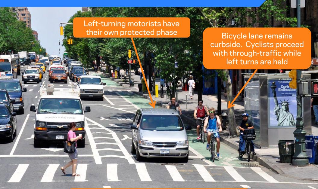
Takes advantage of the existing left turn signals at E 57<sup>th</sup> St and E 59<sup>th</sup> St intersections
