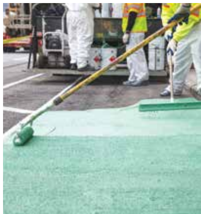
Application of green MMA to bicycle lane
