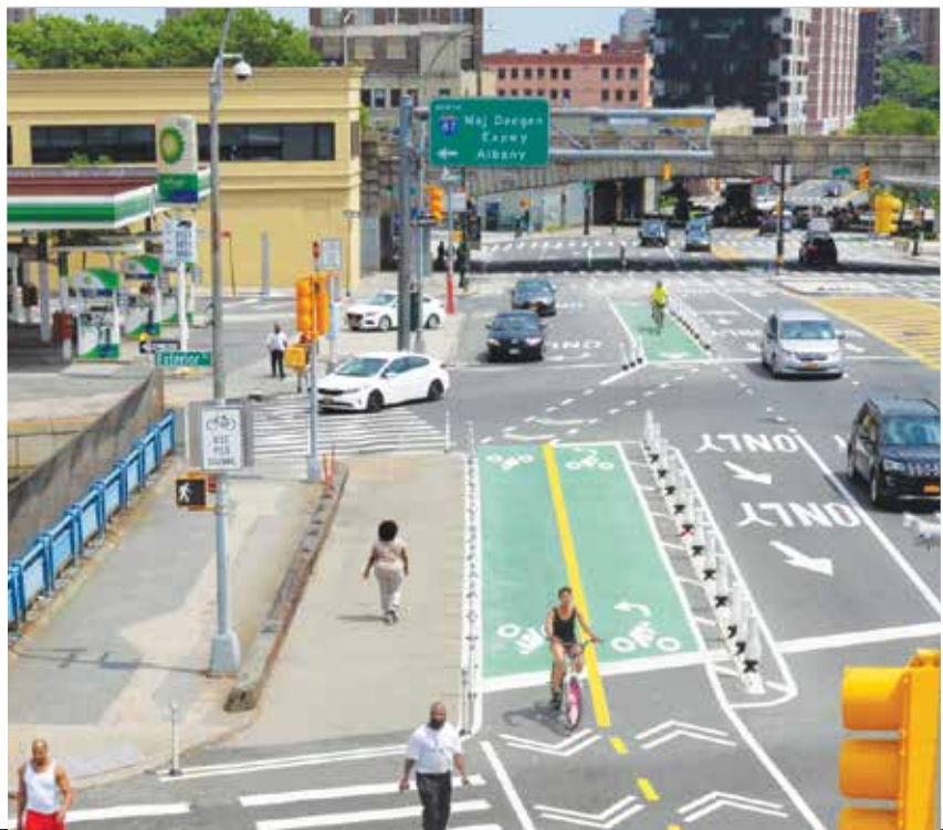
Protected Bicycle Connection with Painted Sidewalk Extension at 138th St in the Bronx
