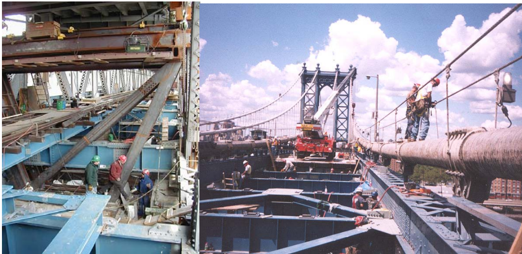
Contract #10 Temporary Truss Jacking Frame Used in the Work to Replace the Existing Truss Bearings. Replacement of Steel Stringers and Floorbeams on the North Upper Roadway Main Span.
