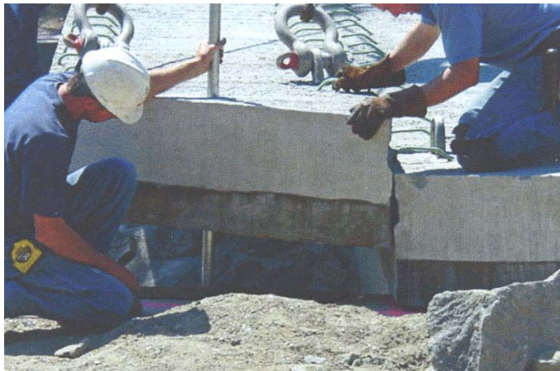
Isham Park – Installation of Precast Slab Panels (Credit: Nasir Khanzada)
