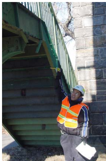
Flag Engineer Inspecting a Yellow Flag (Loose Masonry Panel) on the BQE under the Brooklyn Bridge (Credit: Andy Hoang)
