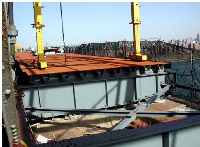
Contract #7 Installing An Orthotropic Deck Panel
