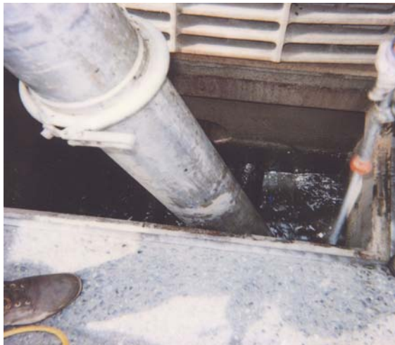
Cleaning Catch Basins on the Manhattan Bridge
