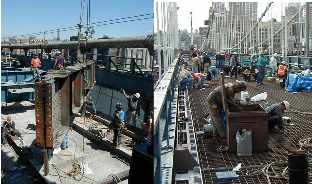
Contract #10 Removing an Existing North Upper Roadway Floorbeam on the Main Span of the Bridge. Installing the New Grid Deck for the North Upper Roadway on the Brooklyn Side Span.
