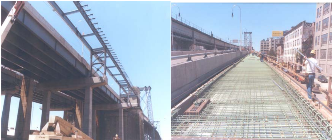
Contract #7 Bikeway Steel Erection & Rebar Installation
