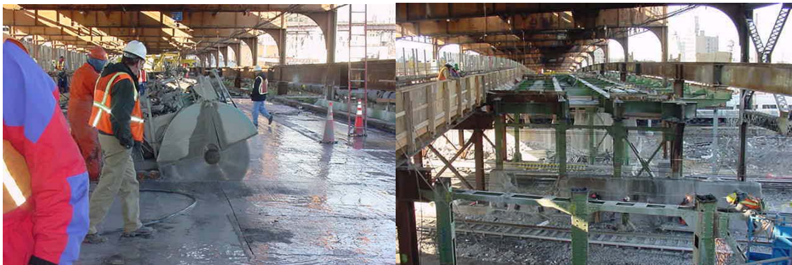
Full Depth Saw Cutting of Queens Boulevard Bridge Deck Slab Panels & Front Steel Demolition
