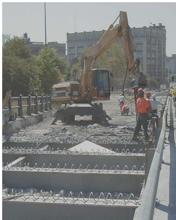
Removal of the Existing Roadway Above the North Subway Tunnel Roof on the Brooklyn Side of the Manhattan Bridge
