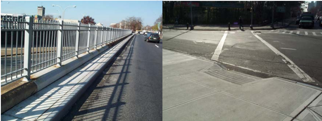
New Curb and Bridge Railing. New Pedestrian Ramp (Credit: Joseph Saverino)
