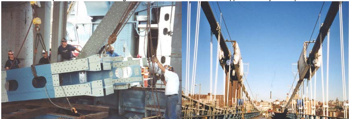
Contract #10 Installing a New End Frame on the Main Span Side of the Brooklyn Tower. Painting Containment Structures on the Cables of the Manhattan Approach Span.
