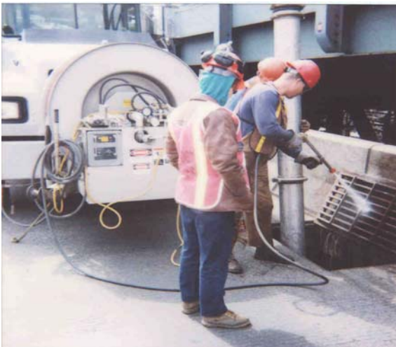
Cleaning Catch Basins on the Manhattan Bridge
