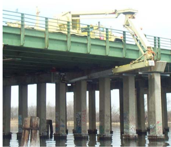
Bridge Inspectors in Snoopers under the Macombs Dam Bridge (Credit: Bojidar Yanev) and the Mill Basin Bridge (Credit: Jyotish Shah)
