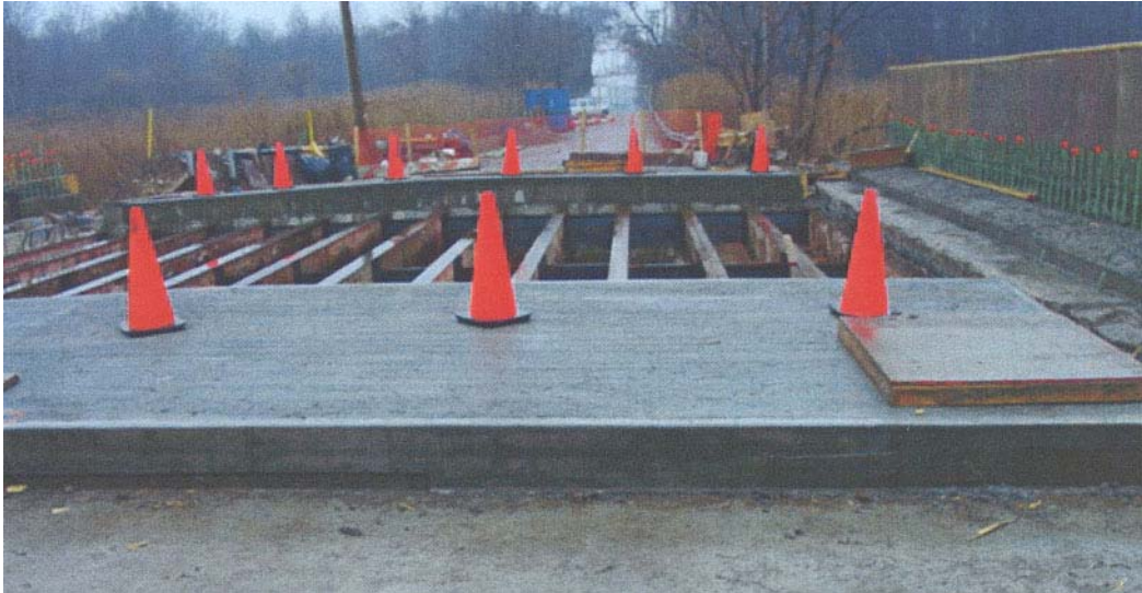
Travis Avenue - Structural Deck and Sidewalk Construction (Credit: Nasir Khanzada)
