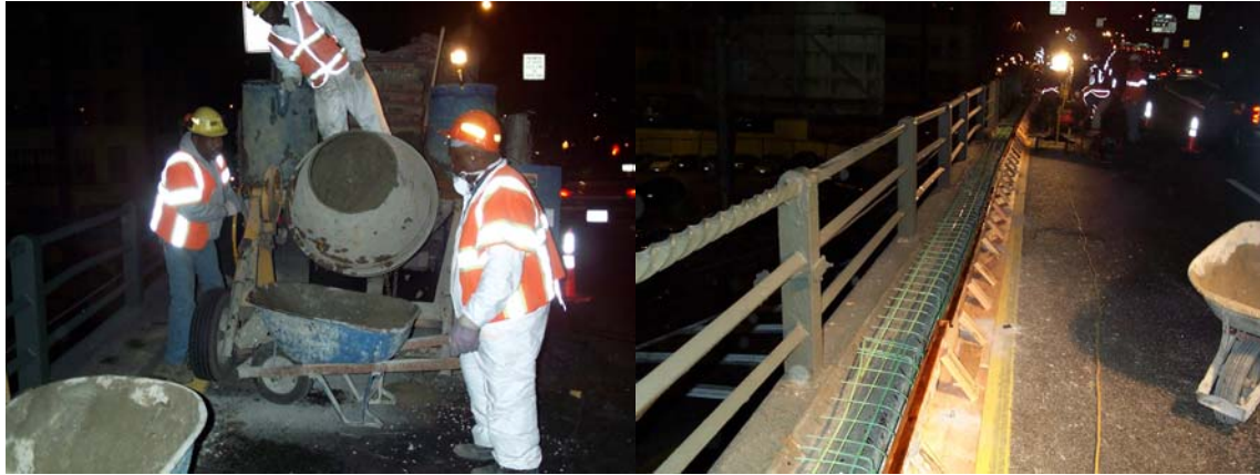
BQE – Batching the Concrete & Form Ready for Concrete (Credit: Joseph Saverino)
