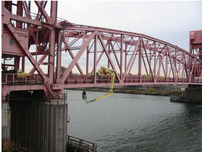
Bridge Inspectors in Snooper Under the Roosevelt Island Bridge (Credit: Bojidar Yanev)
