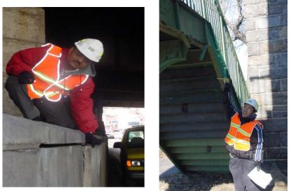
Flag Engineer Inspecting a Yellow Flag (Loose Masonry Panel) on the BQE under the Brooklyn Bridge (Credit: Andy Hoang) Flag Engineer Inspecting a Yellow Flag (Bottom Flanges are Corroded and Loose) at the Inwood Hill Park Footbridge (Credit: Tiffany Yau)
