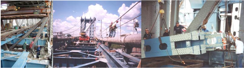
Contract #10 Temporary Truss Jacking Frame Used in the Work to Replace the Existing Truss Bearings. Replacement of Steel Stringers and Floorbeams on the North Upper Roadway Main Span. Installing a New End Frame on the Main Span Side of the Brooklyn Tower.
