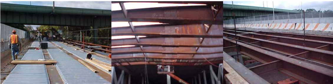
Installation of Stay-in-Place Deck Forms on the 2 nd Avenue Bridge. Structural Steel Erection.
