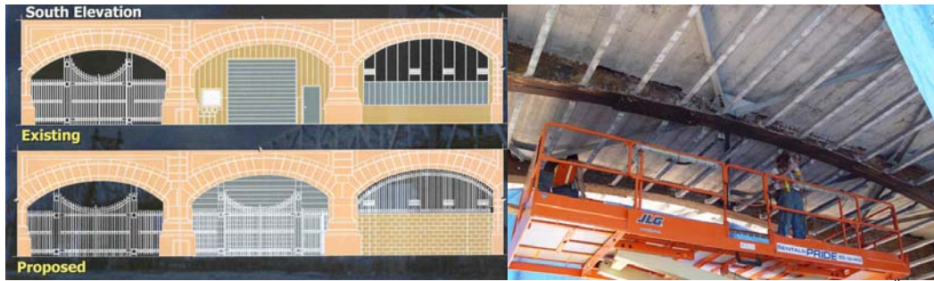
Proposed Rehabilitation of the Arch Infill for the Sanitation Department. Repairing the Steel of the 59 th Street Arch Ceiling.
