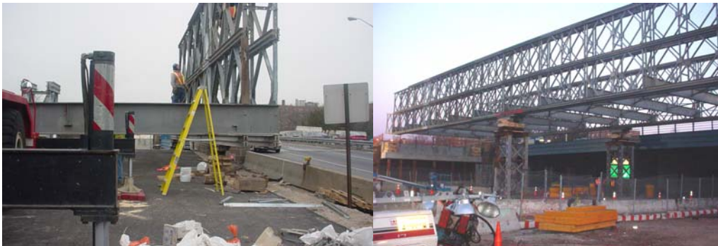
Assembling the Temporary Bridge. Nose of the Temporary Bridge Nearly at the West Abutment. (Credit: Valeriya Remezova)
