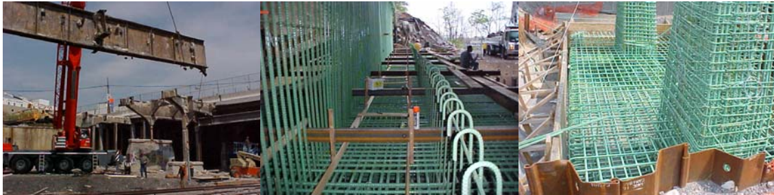
Demolition of the 2 nd Avenue Bridge Superstructure. Abutment Footing and Stem Reinforcement. Installation of Footing and Column Reinforcement for the Bridge's Center Pier.
