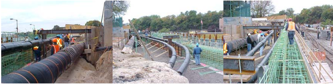
Installation of Safety Wrap Around the High Pressure Gas Main and the Con Edison Oil-o-Static Pipeline. Installation of Reinforcement in the 7 th Avenue Bridge Abutment Stem and Backwall.
