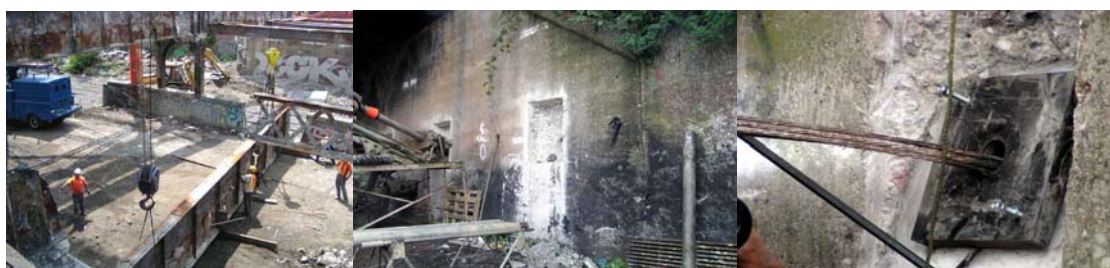
Demolishing the Old Glenmore Avenue Bridge. Installing Tiebacks at the East Abutment.
