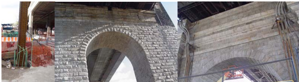
NYCT Column Relocation Work. Anchor Pier Granite Cleaning in Progress.
