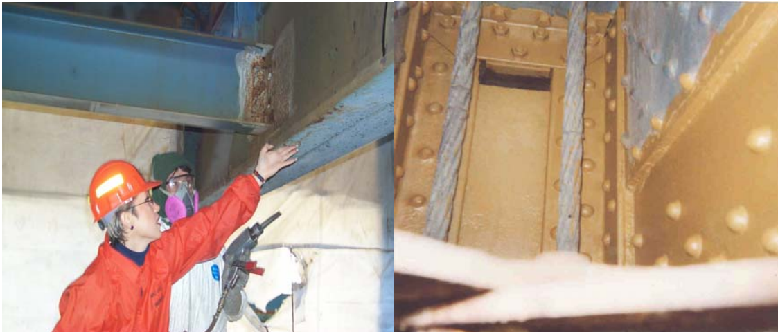
Spot Cleaning Before Painting on the Williamsburg Bridge. Primer Coating on the Williamsburg Bridge.
