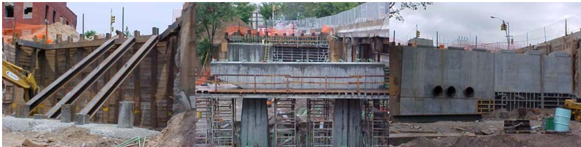
Excavation Protection System at the New 2 nd Avenue Bridge North Abutment. View of the Partially Completed Center Pier and South Abutment. View of the New North Abutment Stem Wall.
