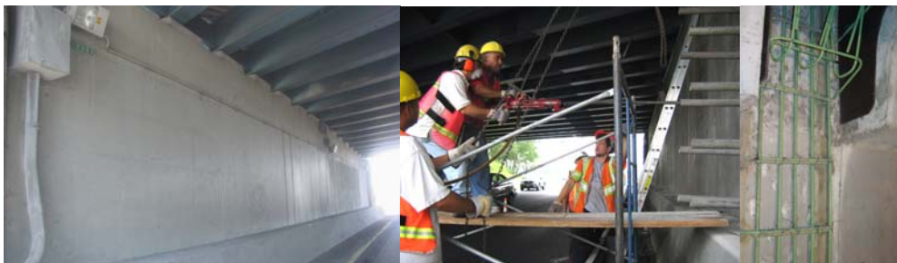
View of the Center Pier Before Project Start. Drilling the Holes at the Center Pier—Assistant City Highway Repairer Robert Rivas, Highway Repairer Vincent Sciulla, Cement Mason John Padovano, & Highway Repairer James Barlett. (Drilling Credit: Peter Basich) Rebars Installed by Ironworkers for Each Buttress.
