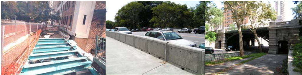
Newly Installed Structural Steel Floor Beams Along the East Sidewalk. Completed Pedestrian Concrete Barrier. Looking East from West 96 th Street at the Newly Rehabilitated Bridge.
