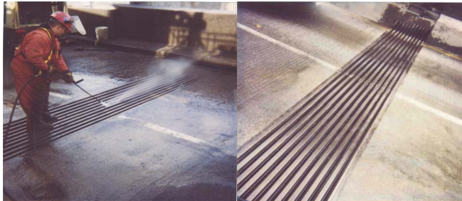
Expansion Joint Cleaning on the Manhattan Bridge. Clean Expansion Joint on the Manhattan Bridge
