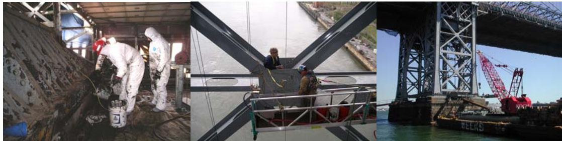
Contract #8 Degreasing the Brooklyn Main Tower Saddle Bearing. Manhattan Main Tower Member Replacement & South Pier Platform Erection.
