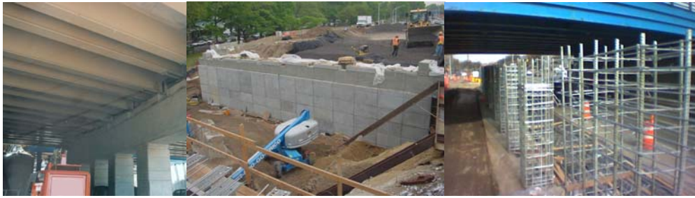
New Stringers Under the Deck and A Pier. Completed Northeast Abutment Retaining T-Wall and Abutment Cap Beam. Reinforcing for the Cast-in-Place Pier Columns.
