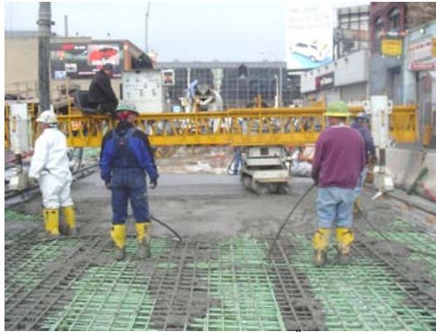
Deck Placement for the West 37 th Street Bridge.
