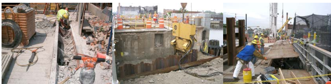
Demolition of the Northwest Flanking Span of the Metropolitan Avenue Bridge. Looking West at the Installation of Sheet Piles on the Northeast Approach Slab. Looking West at the Removal of the Northwest Sidewalk.
