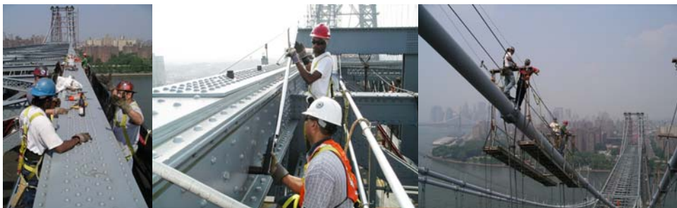
Looking West at the North Truss Top Chord Steel Rehabilitation. High Strength Bolt Torque Inspection. Cable Band Bolt Retensioning.
