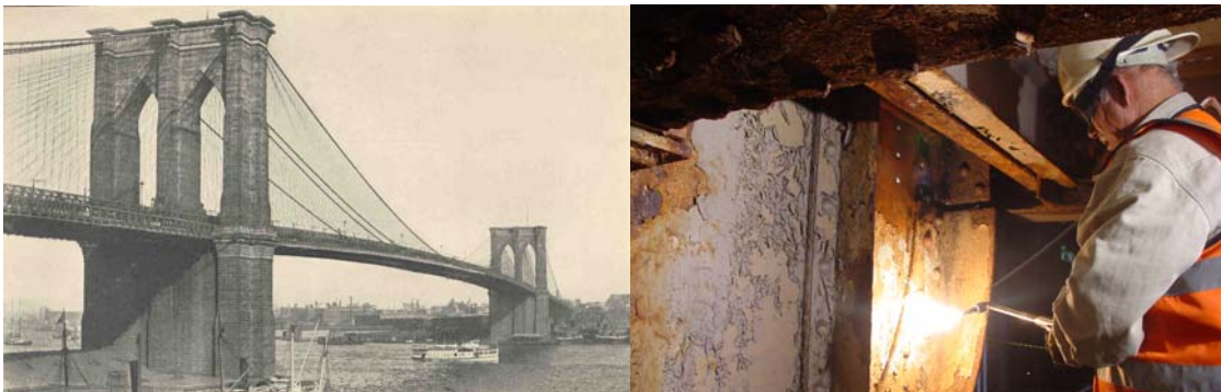
Brooklyn Bridge in 1909. Bridge Repairer & Riveter Joseph Antony Repairing a Red-Flagged Stringer on the Bridge. (Repair Credit: Hany Soliman)
