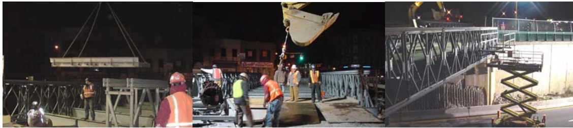
Erection of the South Temporary Bridge.
