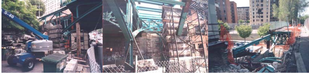
View of the Bridge Under Construction Showing the Marked Granite Stones to be Reinstalled. Newly Installed Structural Steel Members Along the East Sidewalk. View of the New Structural Steel Fascia Girder Being Installed.
