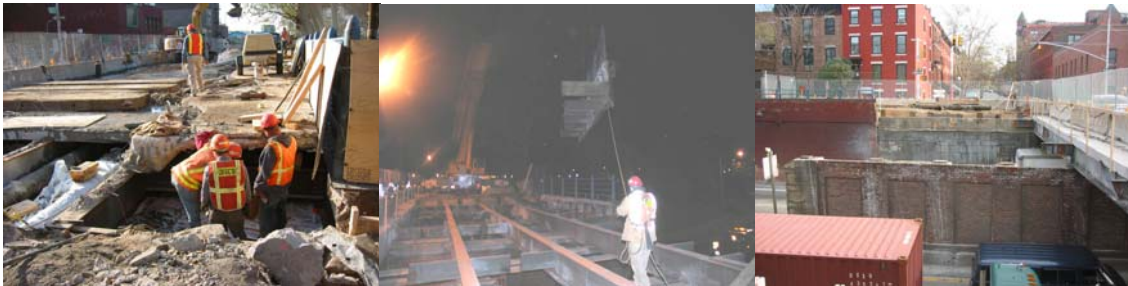
Congress Street Bridge Deck Demolition and Structural Steel Removal. (Credit: Carlos Ramirez)
