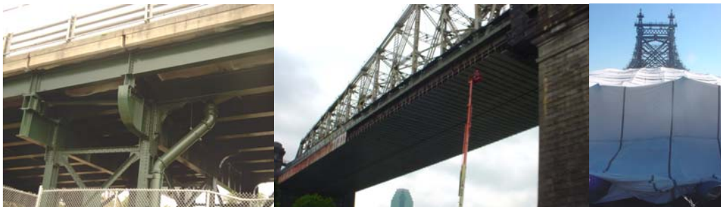
Detail of Freshly Painted East 241 st Street Bridge. Queensboro Bridge Work Platform & Containment. (Queensboro Credit: Daniel Lima)
