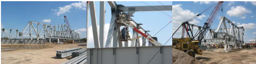
South Truss of New Third Avenue Swing Span Fully Erected in Alabama in March 2004. Installation of Top Lateral Bracing. Erecting the Northeast Section of the Truss. (Credit: Rahul Shah)
