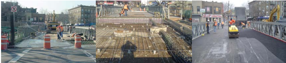
Concrete & Asphalt Work on the Temporary Bridges.
