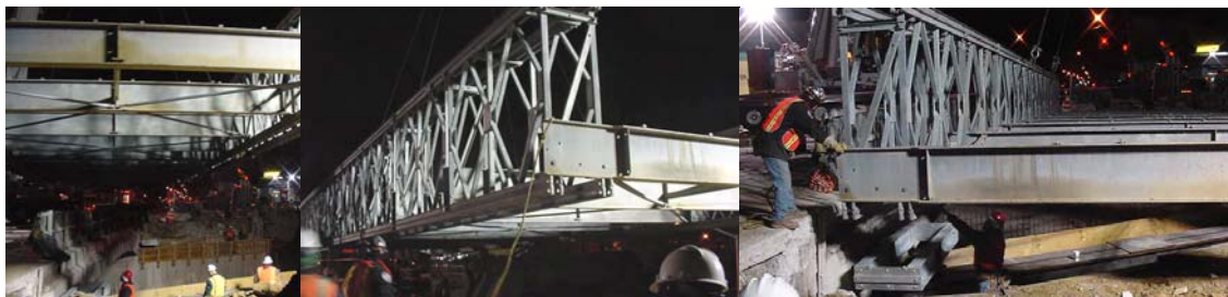
Erection of the North Temporary Bridge.
