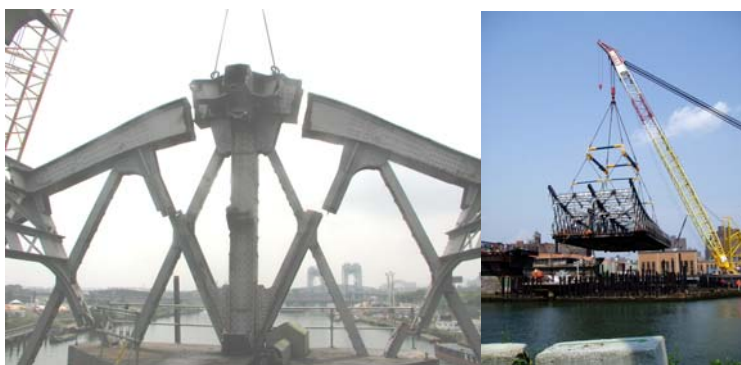
Starting the Removal of the Old Swing Span. Removing the Bronx Half of the Old Swing Span. (Credit: Daniel Hom)
