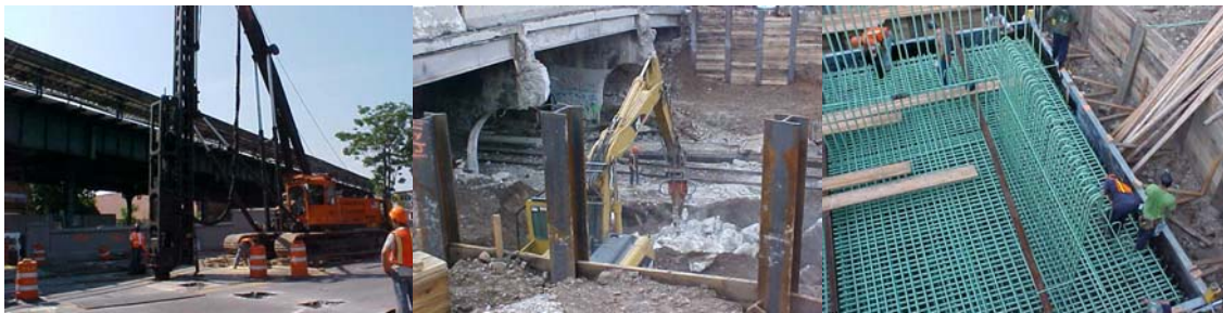
Installation of the Soldier Piles for the Excavation Protection System for the 14 th Avenue Bridge. Excavation for the Abutment Footing. Installation of Abutment Footing.
