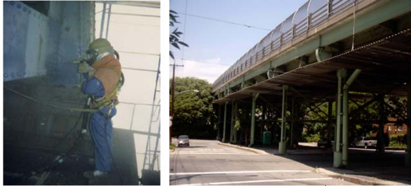
Abrasive Blasting. Platform Installed for Painting of the East 241 st Street Bridge.
