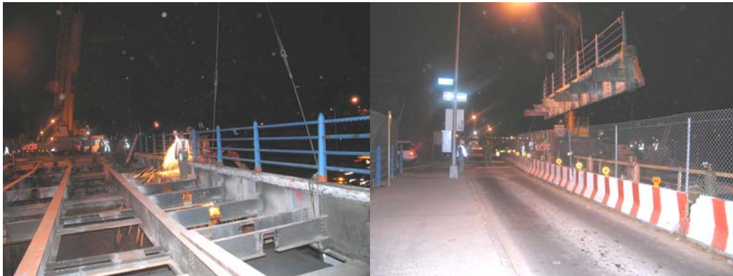
Structural Steel Removal on the Congress Street Bridge. (Credit: Carlos Ramirez)
