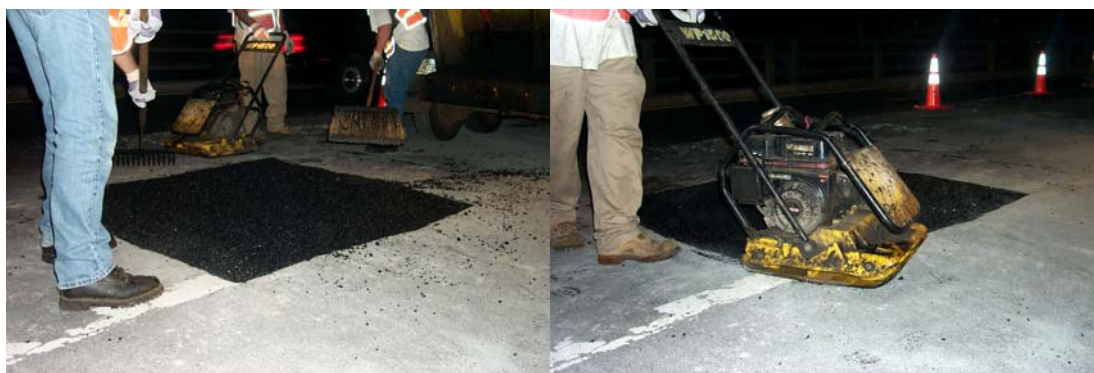
Rolling and Tamping the Asphalt on the Eastbound BQE. (Credit: Anthony Napolitano)
