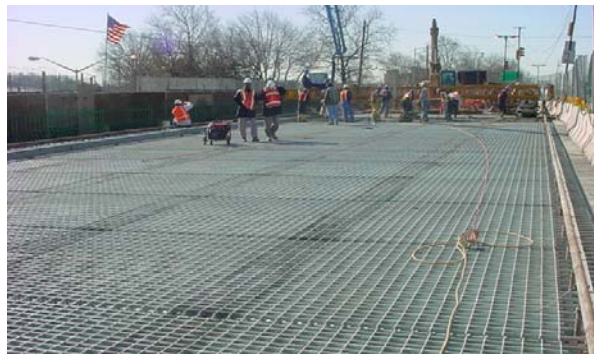
Concrete Placement for the Cross Bay Boulevard Grid Deck.
