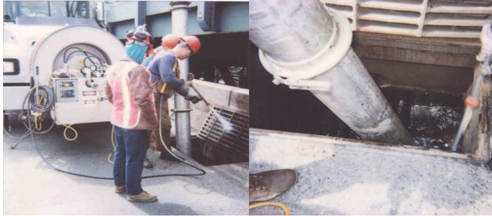
Cleaning Catch Basins on the Manhattan Bridge
