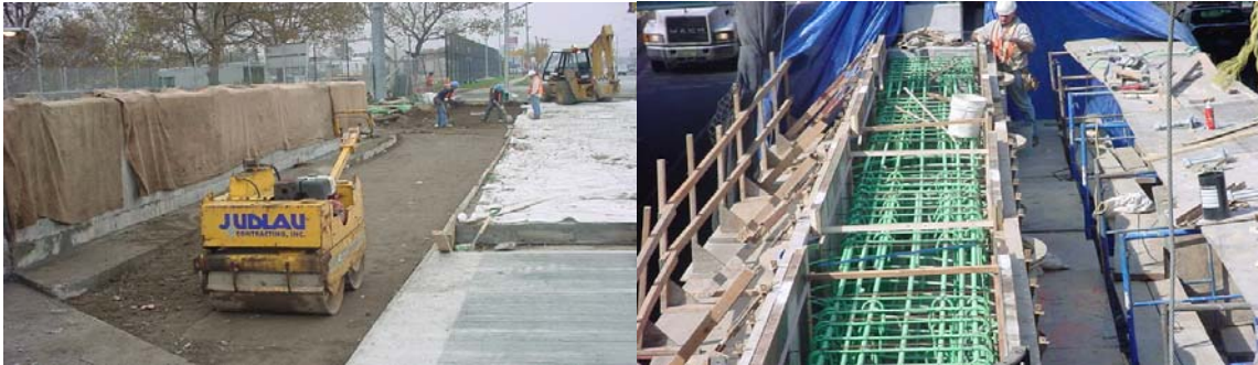
Backfilling and Compacting the Northwest Sidewalk. Curing the Northwest Wingwall and South Roadway. (Credit: Muhammad Siddiqui) Fixing the Formwork During Construction of the Eastern Pier Columns and Cap.
