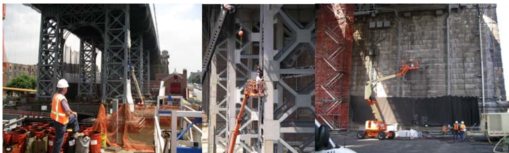
Steel Bracing Replacement Operation at the Brooklyn Intermediate Towers. Ironworkers Bolting up New Steel on Intermediate Tower. Cleaning the Brooklyn Anchorage Exterior Granite Surface.
