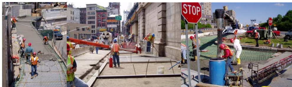
Placing Concrete on Manhattan Approach Ramp of New North Bikeway. Finishing Concrete for the Sidewalk Along Forsyth Street. Engineer-in-Charge Reza Lotf (in White Hard Hat) Inspecting the Placement of Concrete for North Upper Roadway at Nassau Street Intersection.
