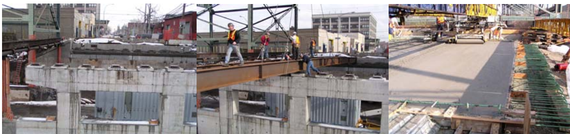
New Bearings Installed at the Central Pier & East Abutment of the Glenmore Avenue Bridge. Erecting Structural Steel. Placing the Deck Slab Concrete.
