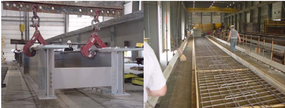
Two Girders For a Precast Unit at the Schuylerville, New York Fabrication Shop. Placing Stainless Steel Reinforcement and Formwork For a Deck Unit at the Shop.
