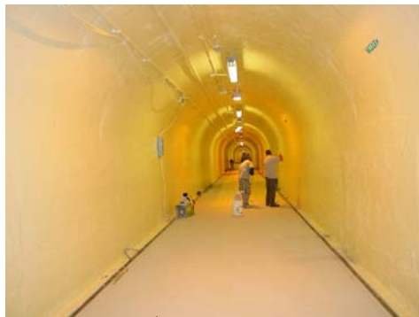
Applying the 2 nd Skid Resistant Coating to the Western Half of the Floor. – the Structure's Lighting Creates the Yellow Tint. (Credit: Thomas Leung)
