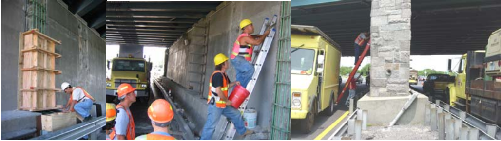
Engineer Hany Soliman Inspecting the Form Work and Rebar Installation Before the Concrete Pour. (Credit: Peter Basich) Cement Masons Frank Finizio, Lawrence Marks, Thomas Valentino, & John Padovano Working on the Pier. (Credit: Peter Basich) Electricians Jerry Salzman & Robert Stackpole Relocating Electric Lines.
