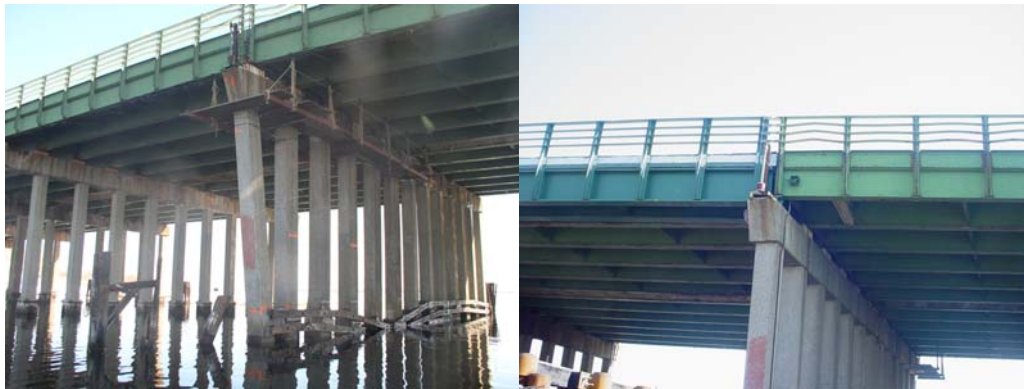
Broken Pier Column at the Belt Parkway Over Paerdegat Basin Bridge in 2003. (Credit: Bojidar Yanev) Connecting Joint of Newly Installed and Existing Span. (Credit: Valeriya Remezova)
