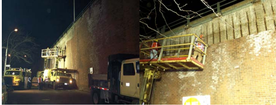
Bricklayers Ignazio Trapani & Salvatore Romano on the Truck Platform Removing the Brick Façade. Cement Masons John Padovano & Thomas Valentino Removing Bricks. (Credit: Joseph Saverino)
