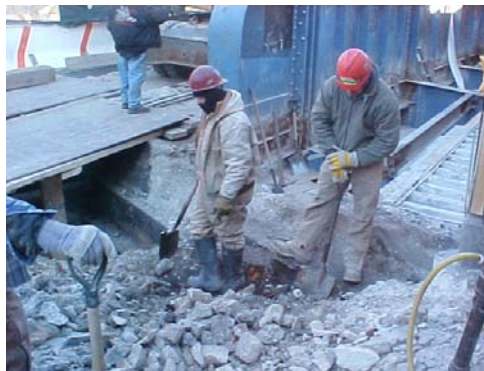
Excavating and Demolishing the Bridge Approach.
