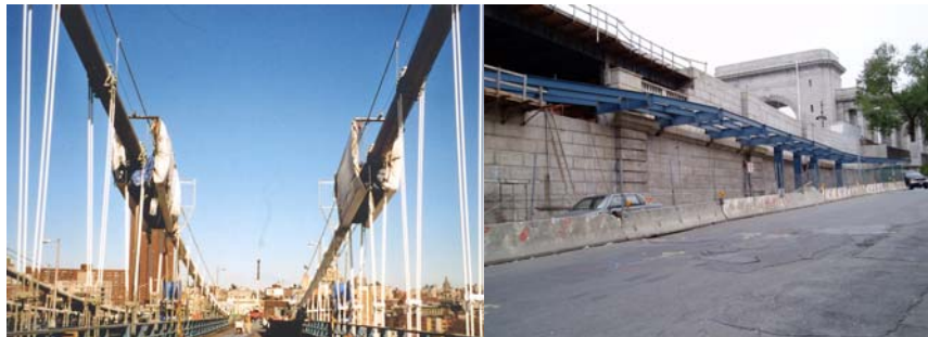
Contract #10 Painting Containment Structures on the Cables of the Manhattan Approach Span. Construction of the New Bikeway Approach Ramp in Manhattan.
