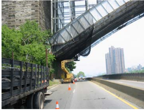
Installing Safety Netting During the Painting of the Washington Bridge. (Credit: Vadim Sokolovsky)
