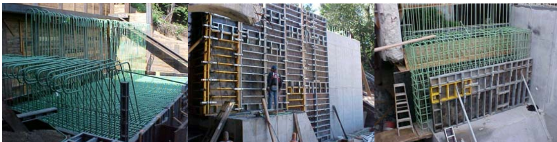
Installation of Stem Reinforcement for the 14 th Avenue Bridge. View of Reinforcement and Form Work Installation at the Bridge Abutment.
