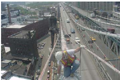
Inspector on Manhattan Bridge Cable. (Credit: NYSDOT)
