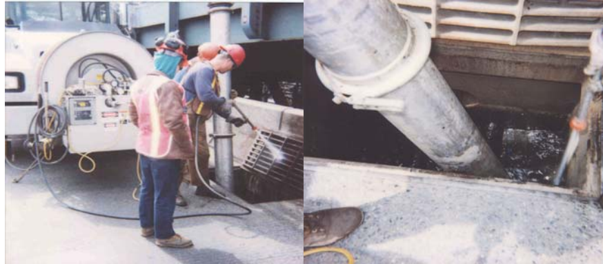
Cleaning Catch Basins on the Manhattan Bridge
