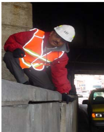
Flag Engineer Inspecting a Yellow Flag (Loose Masonry Panel) on the BQE under the Brooklyn Bridge. (Credit: Andy Hoang)
