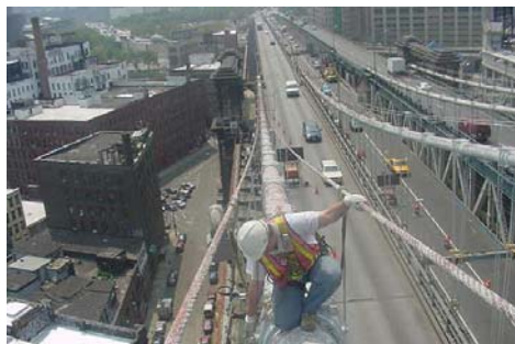
Inspector on Manhattan Bridge Cable. (Credit: NYSDOT)
