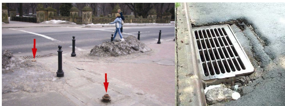
72 nd Street Cross drive Near Concert Grounds – The Posts Were Missing, Leaving the Bases Protruding Above the Sidewalk. This was a Tripping Hazard. Gun Hill Road over Bronx Boulevard – the Asphalt Surrounding the Catch Basin Had Settled, Causing the Grating to Deflect Under Heavy Traffic Loads. This was a Safety Hazard to Vehicles. (Description & Credit: NYSDOT)
