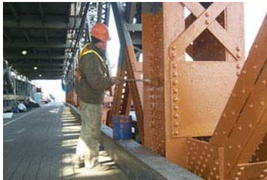
Salt Splash Painting on the Williamsburg Bridge. (Credit: Fouad Althaibani)
