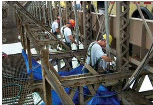
Maintenance Crew Conducting the Annual Cleaning and Lubrication of the Solid Rod Suspenders Spherical Bearings on the Brooklyn Bridge. (Credit: Anatoly Orlov)
