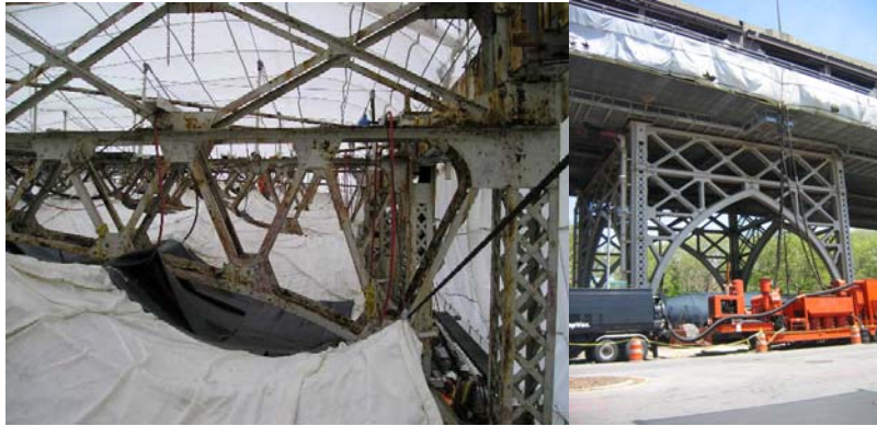
Inside the Queensboro Bridge Containment. Roadway Containment. (Roadway Credit: Michele N. Vulcan)
