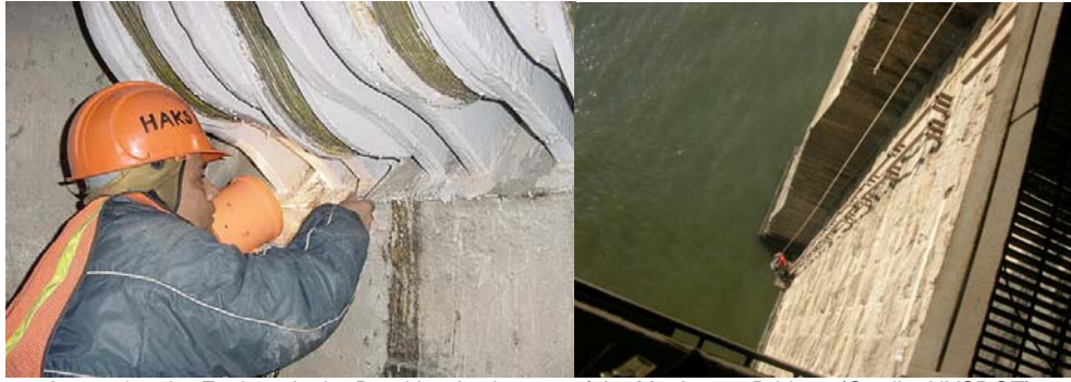
Inspecting the Eyebars in the Brooklyn Anchorage of the Manhattan Bridge. (Credit: NYSDOT) Repairing the Brooklyn Bridge Standpipe System, 130 Feet Below the Roadway.
