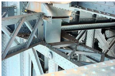
Truss Bearing on Manhattan Bridge. (Credit: NYSDOT)
