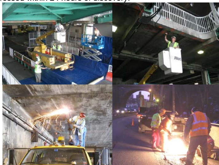
Executive Director of Bridge Preventive Maintenance and Repair Tom Whitehouse (White Hardhat) Ensuring the Proper Setup of Containment Procedures at the St. George Ferry Terminal Landing Slips Before the Masons Address A PIA Flag (Falling Concrete). Inspecting the Flagged Condition. PIA Flag (Truck Wedged Under the FDR Drive at Span 41): Removing the Debris. (Credit: Victor Sandoval) PIA Flag Repair (Through Hole) on Harlem River Drive Ramp. (Credit: Bojidar Yanev)
