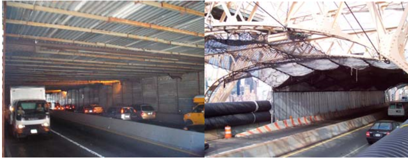
2007 Queensboro Bridge Lower Level and Upper Level Shielding.
