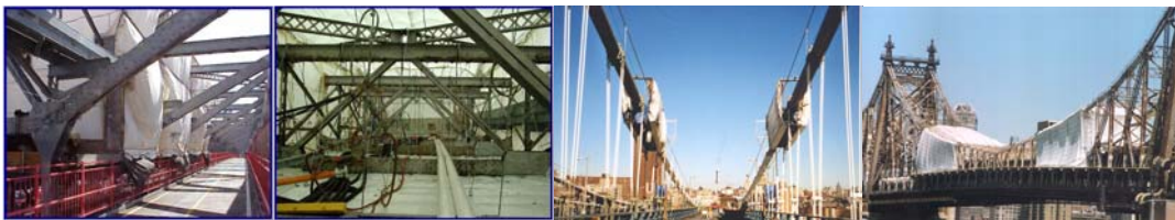
Containment Examples. Manhattan Bridge - Painting Containment Structures on the Cables of the Manhattan Approach Span. 2005: Queensboro Containment. (Queensboro Credit: Peter Basich)
