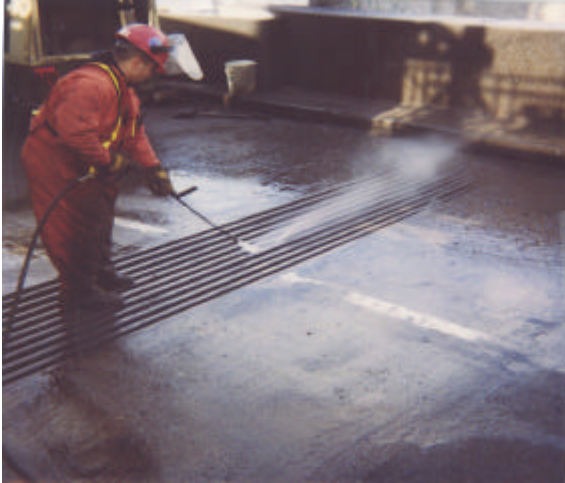
Expansion Joint Cleaning on the Manhattan Bridge
