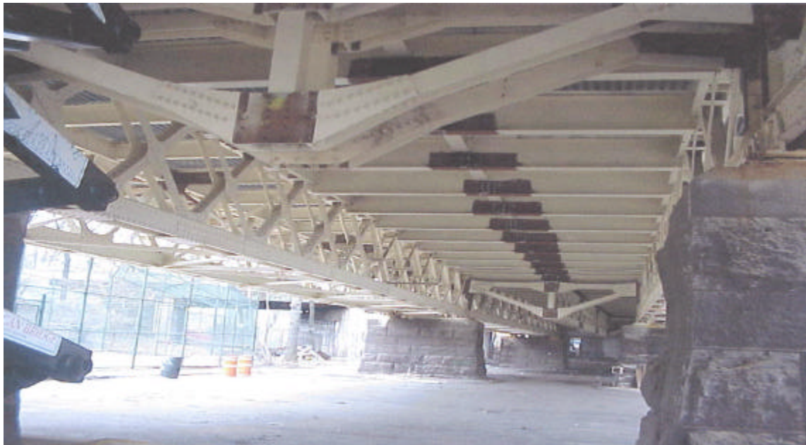
New Trusses at the Jerome Avenue Approach To the Macombs Dam Bridge
