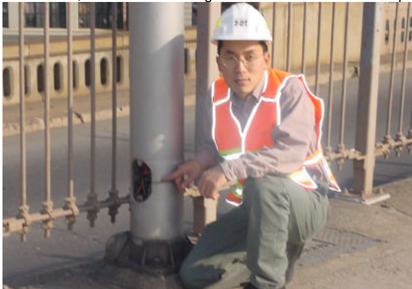
Flag Engineer Inspecting a Safety Flag (Exposed Electrical Wiring) on the Brooklyn Bridge Promenade.
