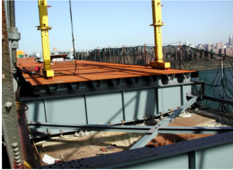
Contract #7 Installing An Orthotropic Deck Panel
