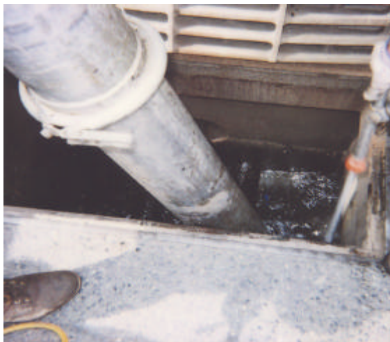
Cleaning Catch Basins on the Manhattan Bridge
