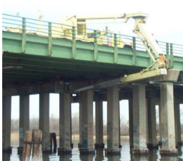
Bridge Inspectors in Snoopers under the Macombs Dam Bridge and the Mill Basin Bridge
