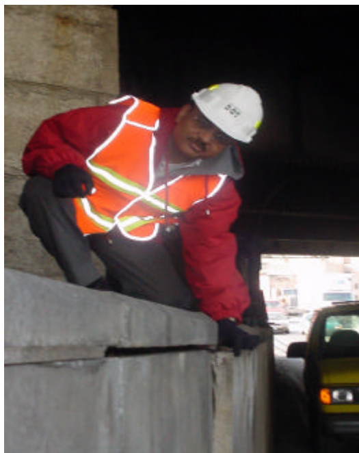
Flag Engineer Inspecting a Yellow Flag (Loose Masonry Panel) on the BQE under the Brooklyn Bridge.
