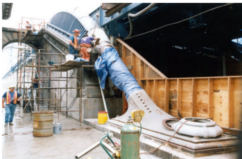
First Saddle Repairs on the Manhattan Bridge Since 1909.
