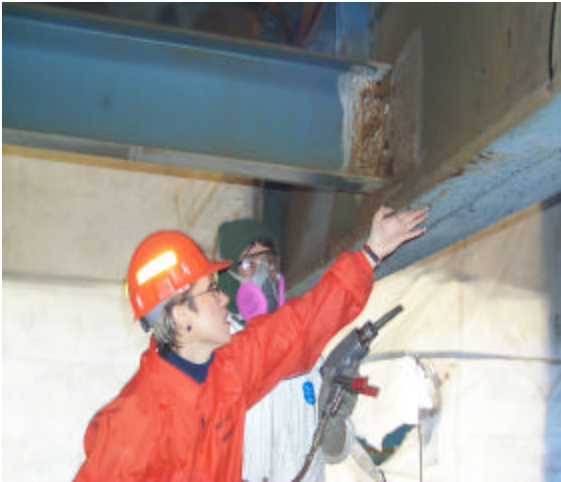
Spot Cleaning Before Painting on the Williamsburg Bridge
