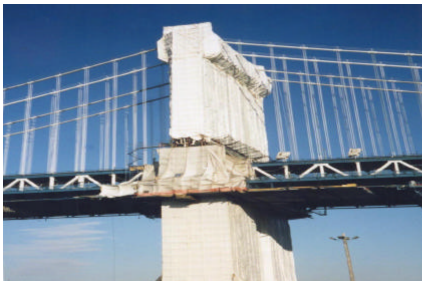
Full Containment on the Manhattan Bridge
