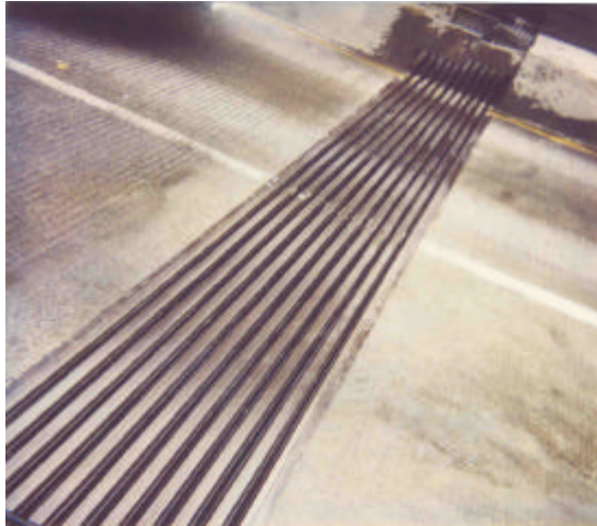
Clean Expansion Joint on the Manhattan Bridge
