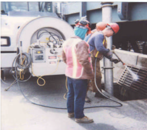
Cleaning Catch Basins on the Manhattan Bridge
