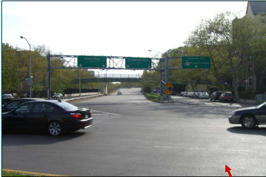
“Expressway” look at ramp
