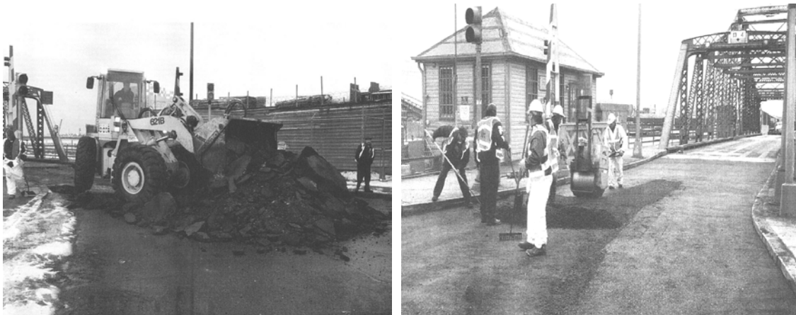
Asphalt Repair on the Grand Street Bridge (Credit: Anthony Napolitano)
