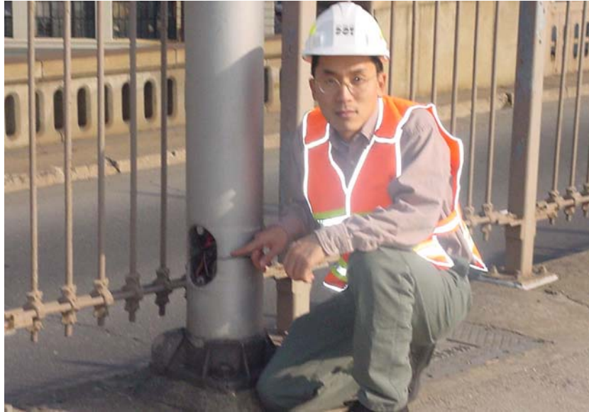
Flag Engineer Inspecting a Safety Flag (Exposed Electrical Wiring) on the Brooklyn Bridge Promenade. (Credit: Rajendra Pandya)
