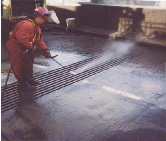
Expansion Joint Cleaning on the Manhattan Bridge
