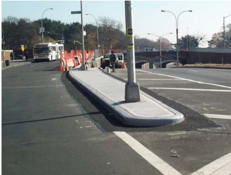
Newly Repaired Bullnose Curb and Sidewalk at Crotona Avenue (Credit: Joseph Saverino)
