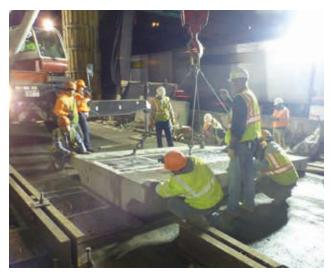
DOT crew installing a Weigh In Motion (WIM) device near the Alexander Hamilton Bridge. These devices collect information about truck weight as vehicles travel on the roadway.
