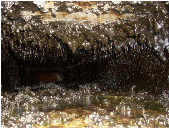
Carbonized, liquid heavy grease
