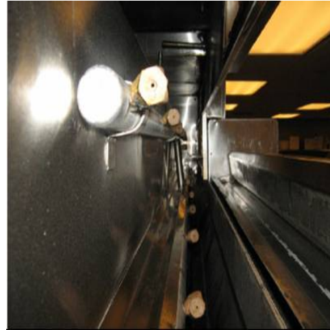
Nozzle installed in a water wash system hood
