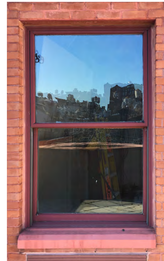
Existing window photo
